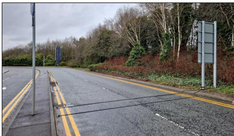
Figure 4-5. Palma Avenue Eastbound ATC - West of Terminal 2 MSCP exit
