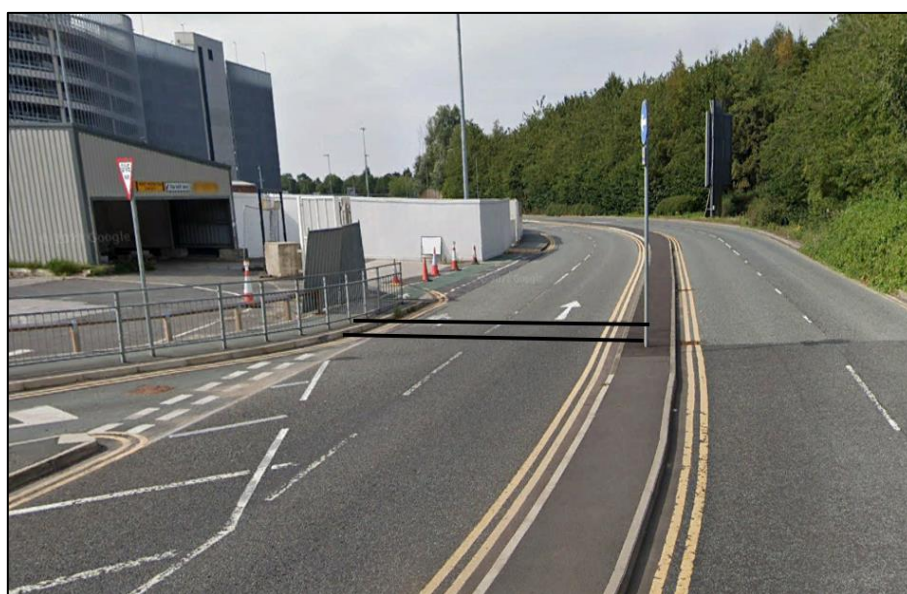
Figure 4-4. Palma Avenue Westbound ATC - West of Terminal 2 MSCP exit
