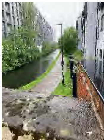
Image 16 – Carruthers Street Lighting Columns (no.21)
