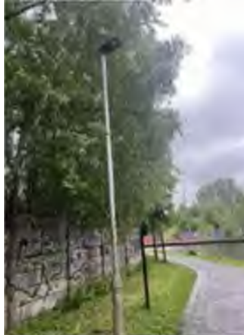
Image 4 – New viaduct Street Lighting Columns (no.33)
