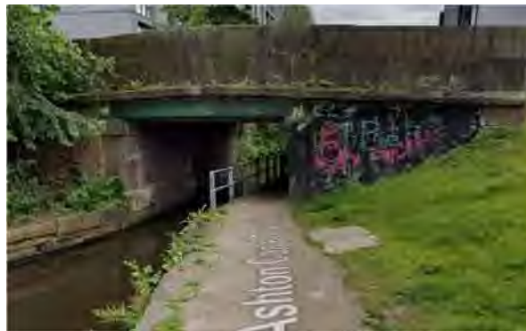
Image 15 – Carruthers Street bridge
