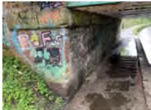
Image 7 – Cambrian Street Bridge
