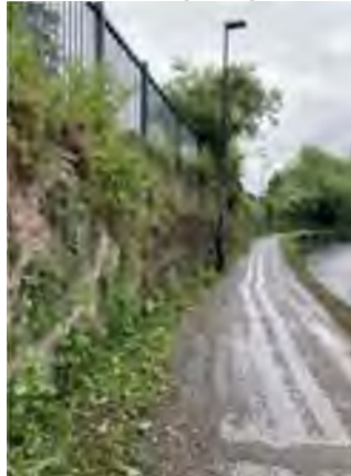
Image 8 – Cambrian Street Lighting Columns (no.34)
