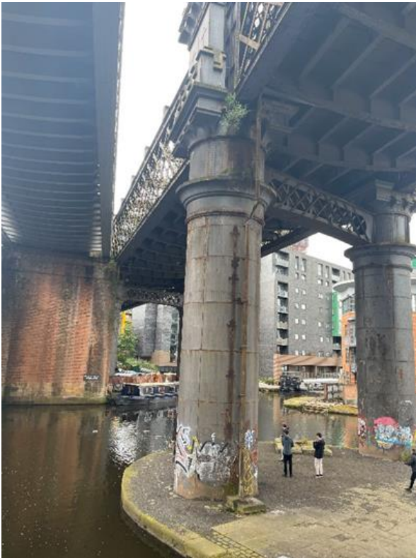
Figure 10 – Castlefield Viaduct Existing Drainage
