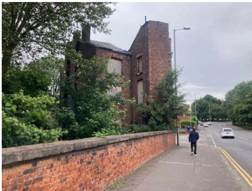
View of building rear from Queens Road
