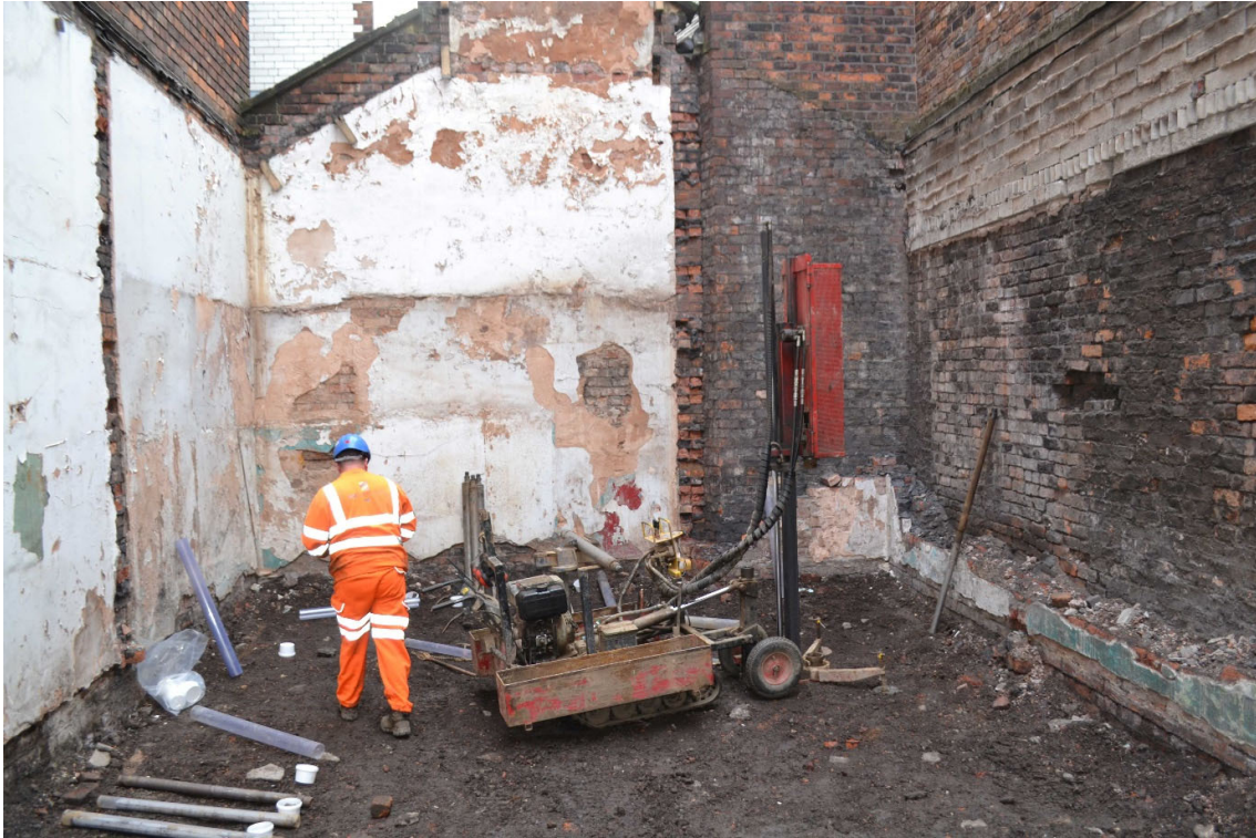
Plate 1: Borehole rig in action
