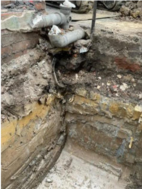
Plate 8: Foundation reception pit sections showing Made Ground surmounting gravelly clay.
