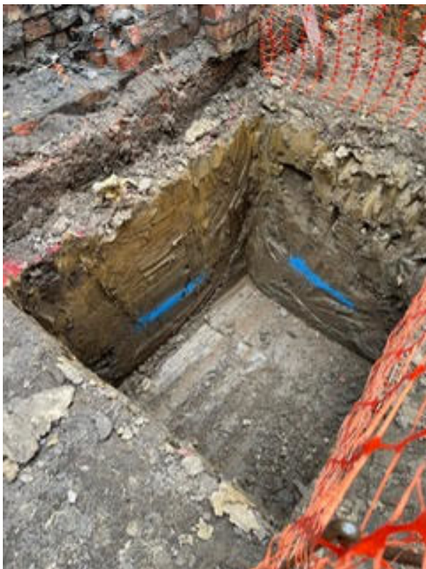
Plate 7: Foundation reception pit sections showing gravelly clay, a geologically lain material consistent in composition with the broad geological definition of Devensian Till
