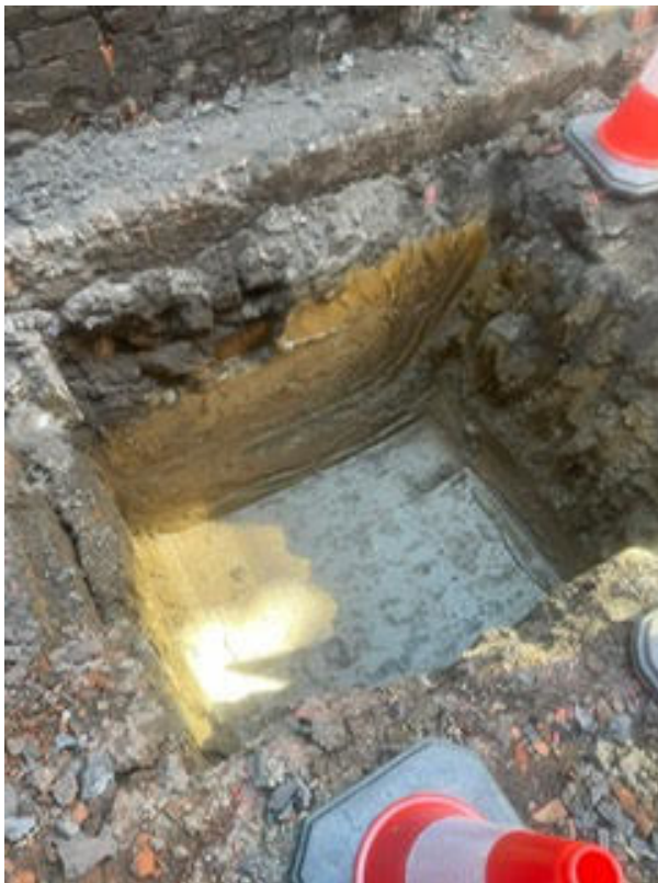
Plate 5: Foundation reception pit sections showing gravelly clay, a geologically lain material consistent in composition with the broad geological definition of Devensian Till
