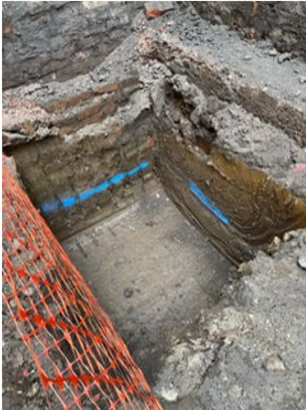
Plate 4: Foundation reception pit sections showing gravelly clay which was a geologically lain material consistent in composition with the broad geological definition of Devensian Till
