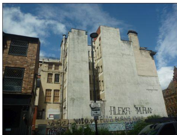
Photo 4: Building 1, southern elevation
