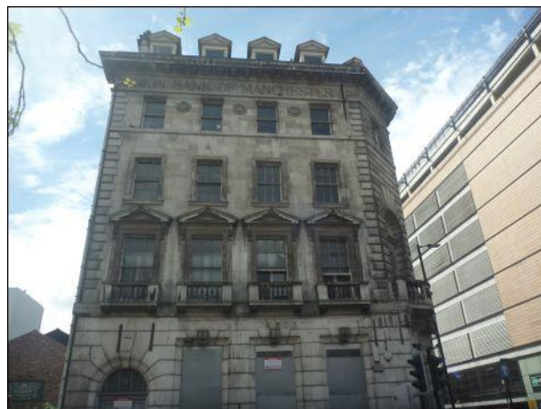
Photo 2: Building 1, eastern (front) elevation
