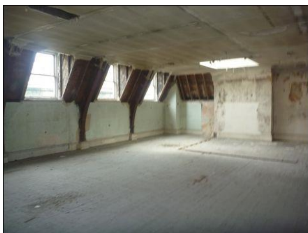
Photo 5: Building 1, internal area, upper floor
