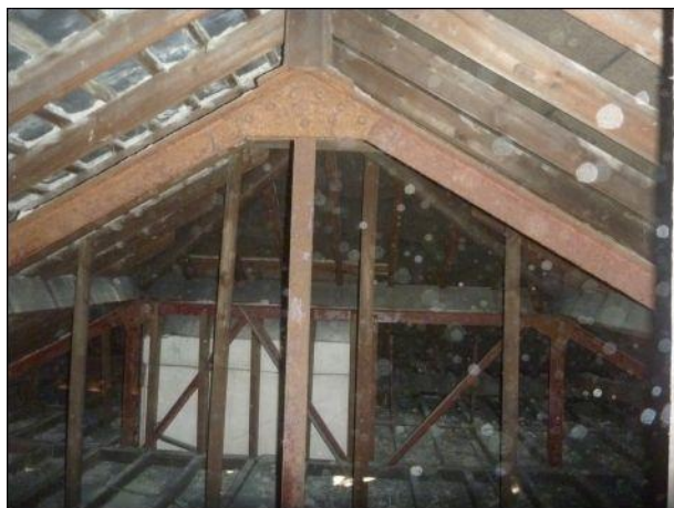
Photo 7: Building 1, roof void
