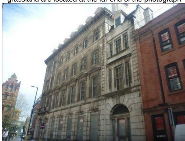
Photo 3: Building 1, northern elevation
