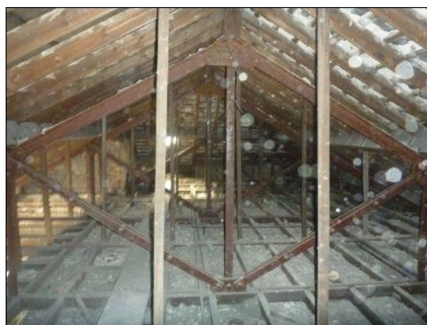
Photo 6: Building 1, roof void
