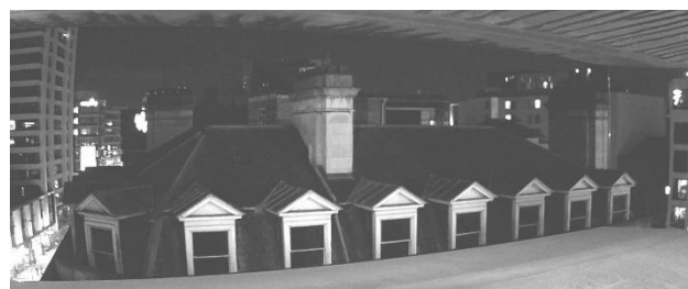
Photo 10: Survey Position 2, facing northern elevation of the building
