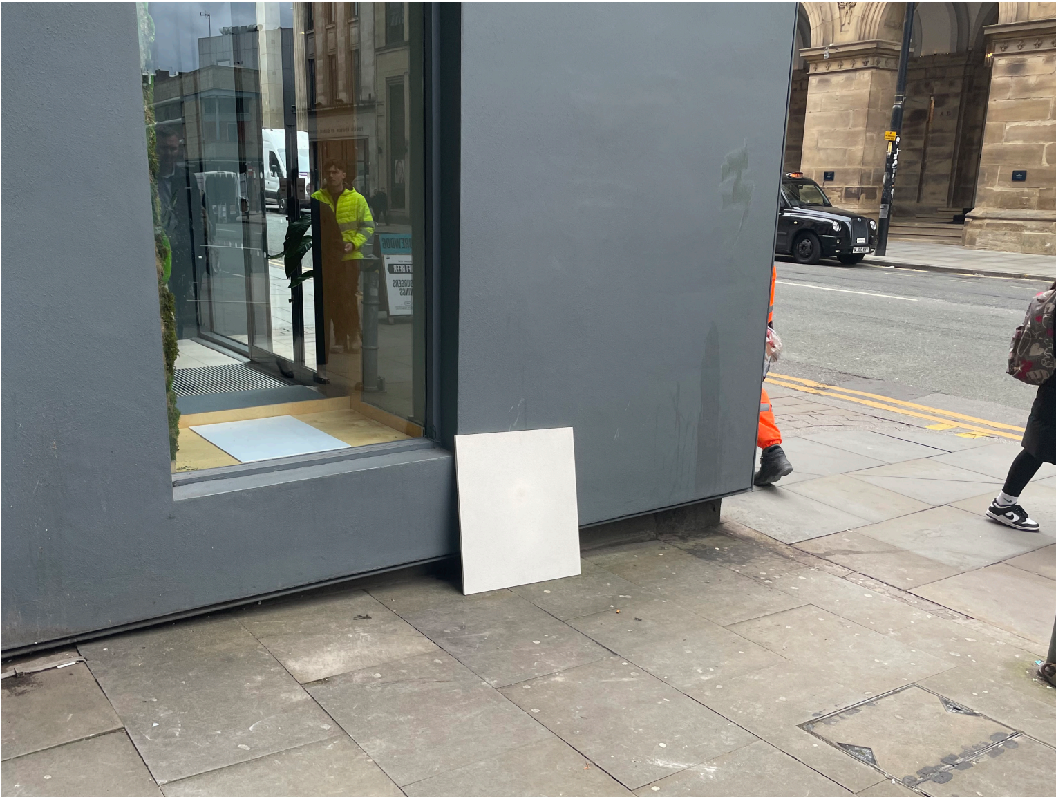
Repaired Sample Panel as viewed externally with MCC 24.05.01
