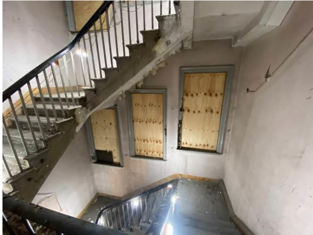
Figure 30: Tiered windows in stair core.
