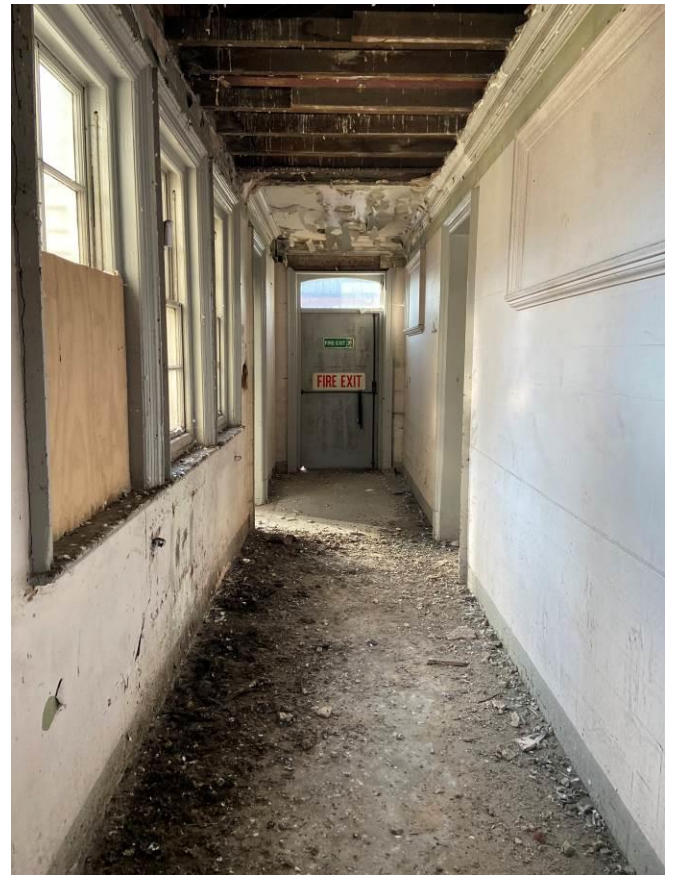
Figure 36: Corridor at upper level leading to external fire escape.
