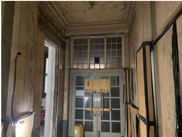
Figure 24: Original timber and glazed doors from Piccadilly entrance into corridor.
