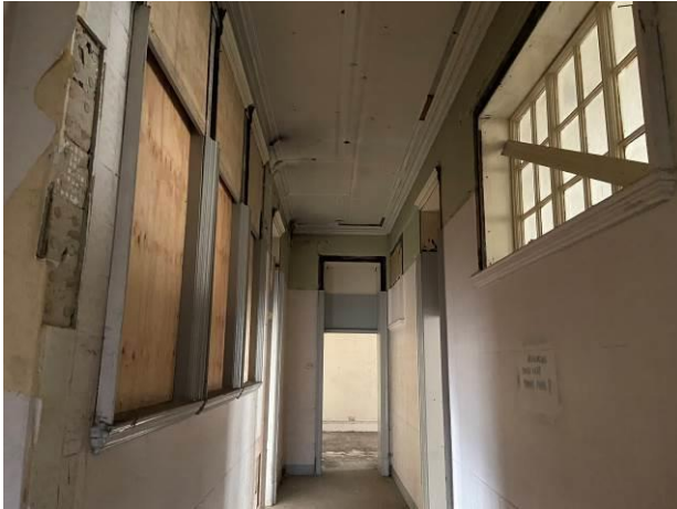
Figure 26: Corridor at upper level with interior windows.
