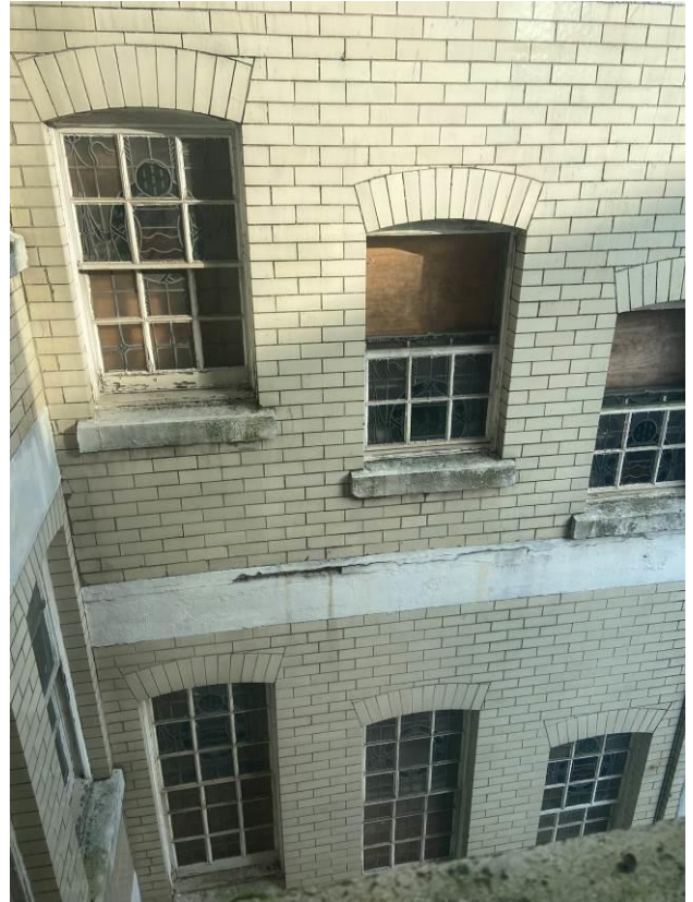
Figure 35: View of stair core from the toilet core including tiered windows with stained and leaded glass and central lightwell.
