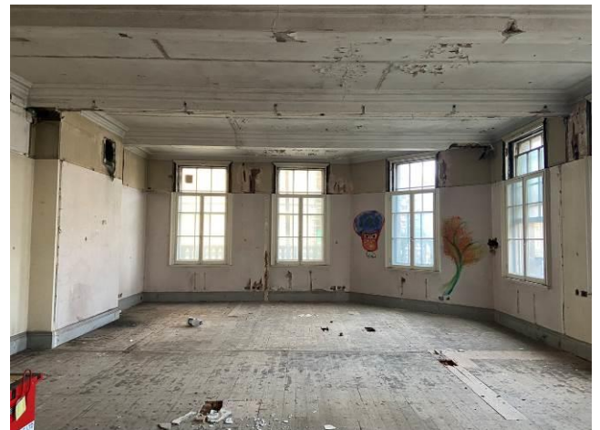
Figure 25: Large room at first floor level with suspended ceiling removed.
