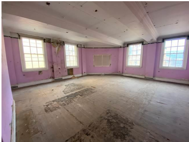
Figure 32: Large room at third floor level with partitions and suspended ceiling removed.
