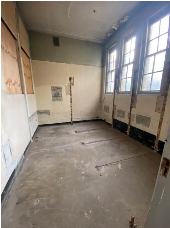
Figure 28: Former toilet block.
