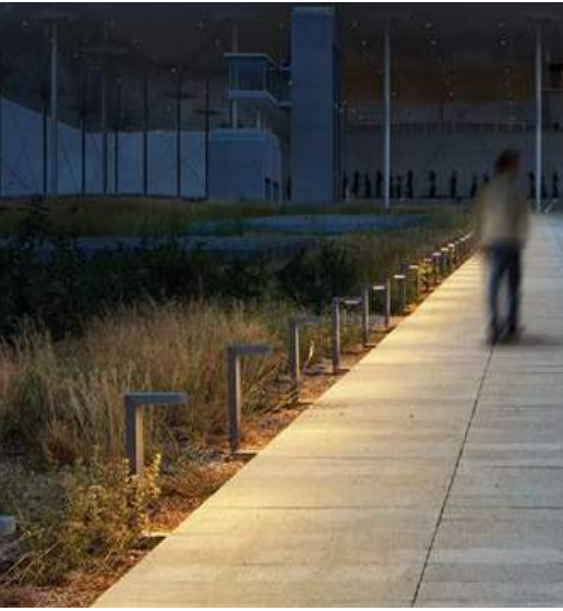
Figure 19: low level bollards to illuminate the walkway
