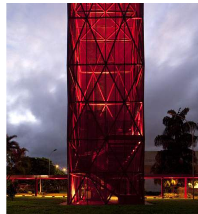
5 Communicate the identity of the viaduct from ground level
