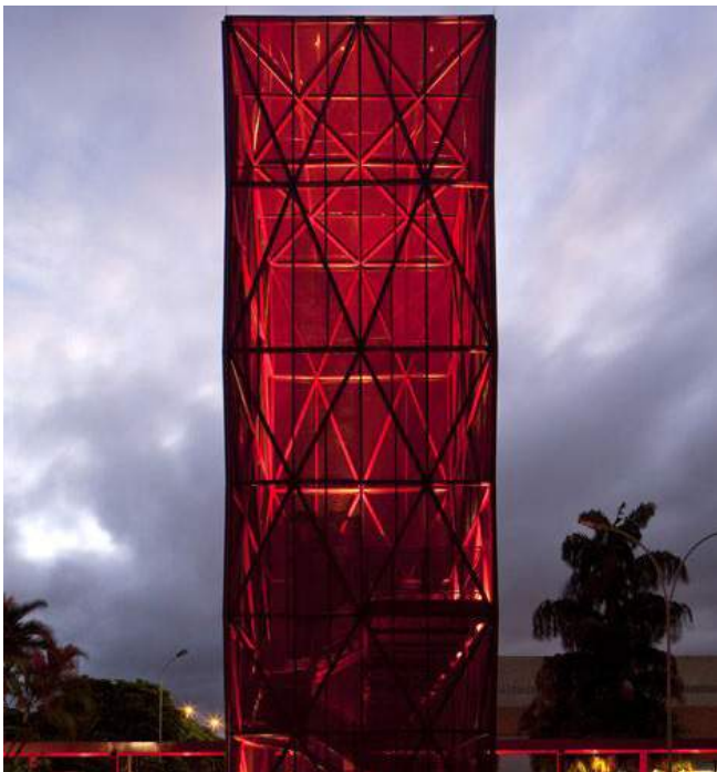
Figure 4: Revealing the structure of the lift and staircase at night
