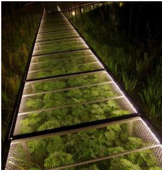
Figure 26: Back-lit mesh walkways
