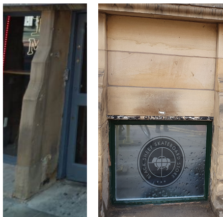
Image 3 - Photo of stoneworks at No.12 and 16 Newton Street to be replicated on the facade of No.10 and 8.
