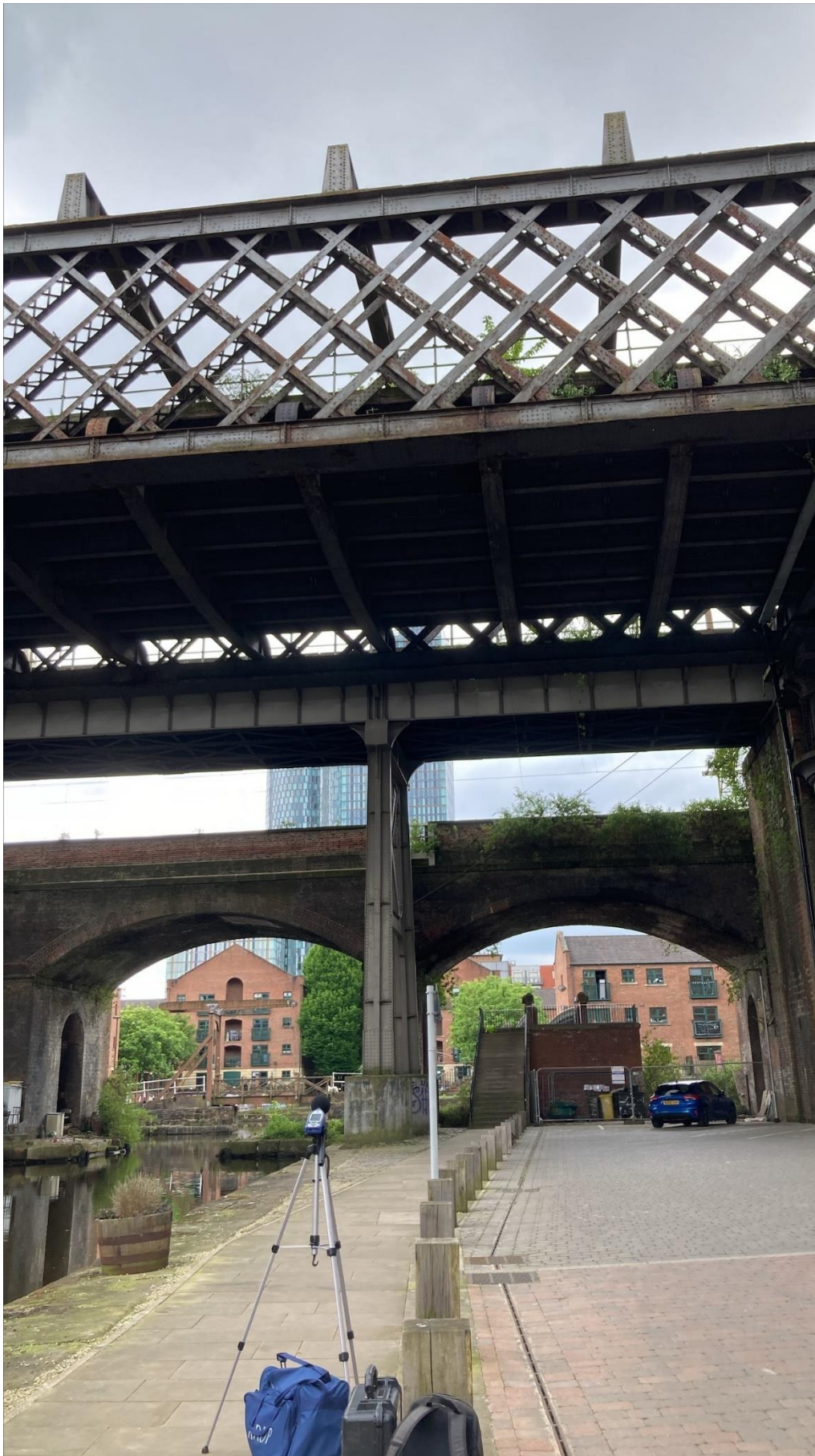
Figure 19: Attended measurement location A4, located at ground level in the centre of the Potato Wharf residential area, facing south towards the viaduct.
