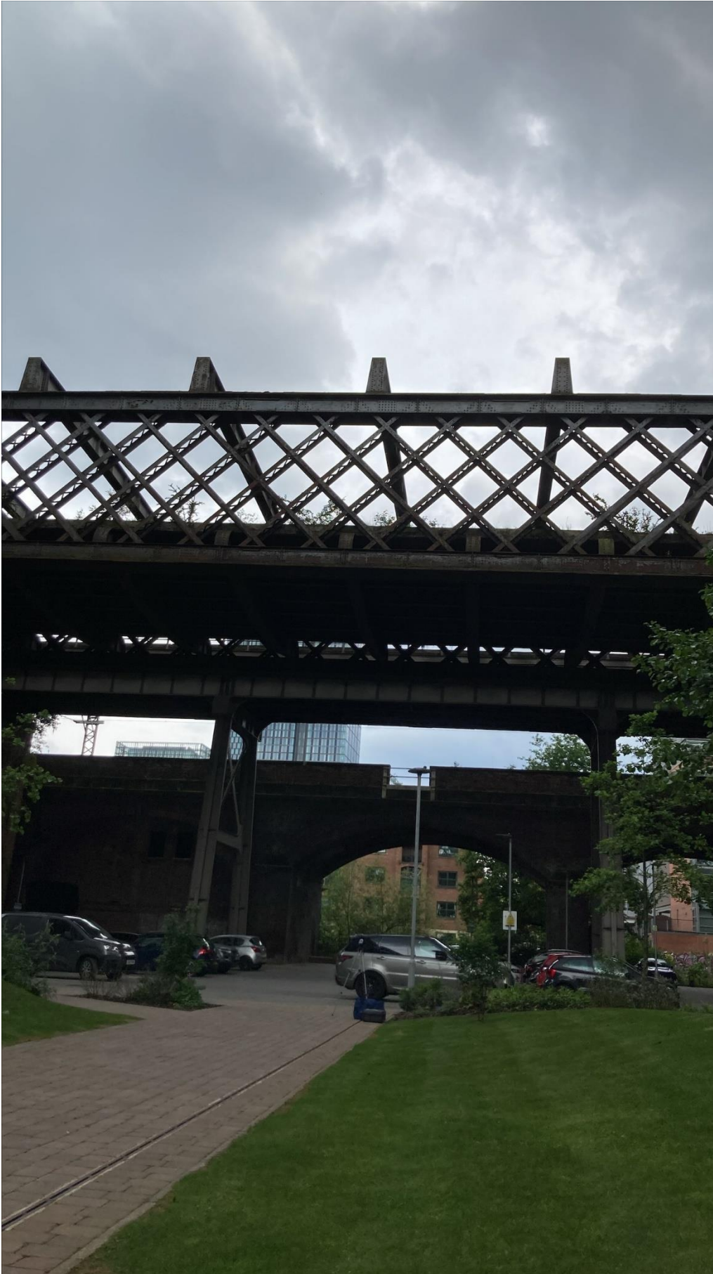
Figure 18: Attended measurement location A3, located at ground level in the centre of the Potato Wharf residential area, facing south towards the viaduct.
