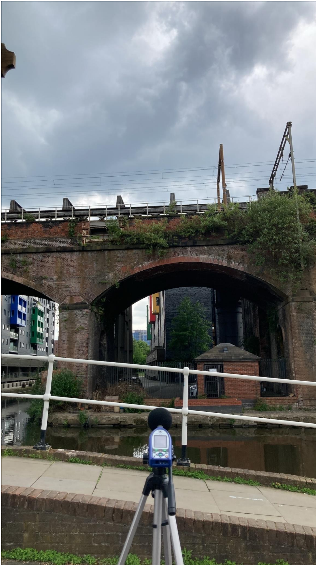
Figure 20: Attended measurement location A5, located at ground level along Bridgewater Canal to the south of Castlefield Viaduct.
