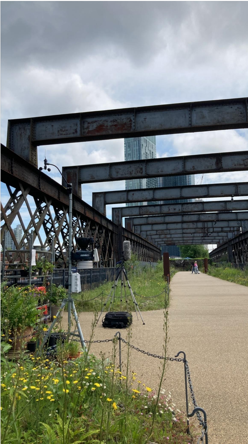
Figure 22: Attended measurement location A6, located in the centre of the existing National Trust viaduct garden.
