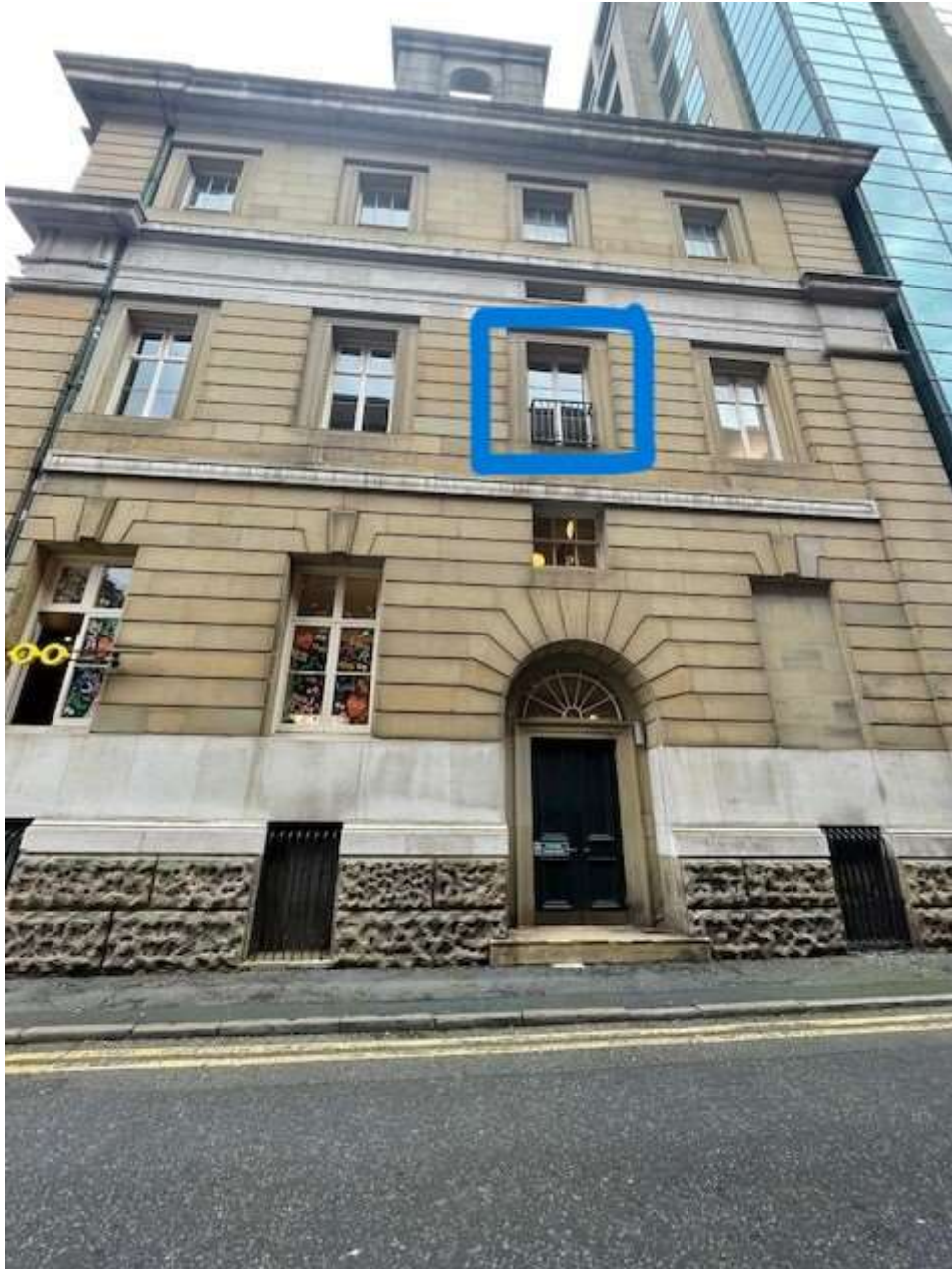
Essex Street Balcony Doors (taken from Essex Street)
