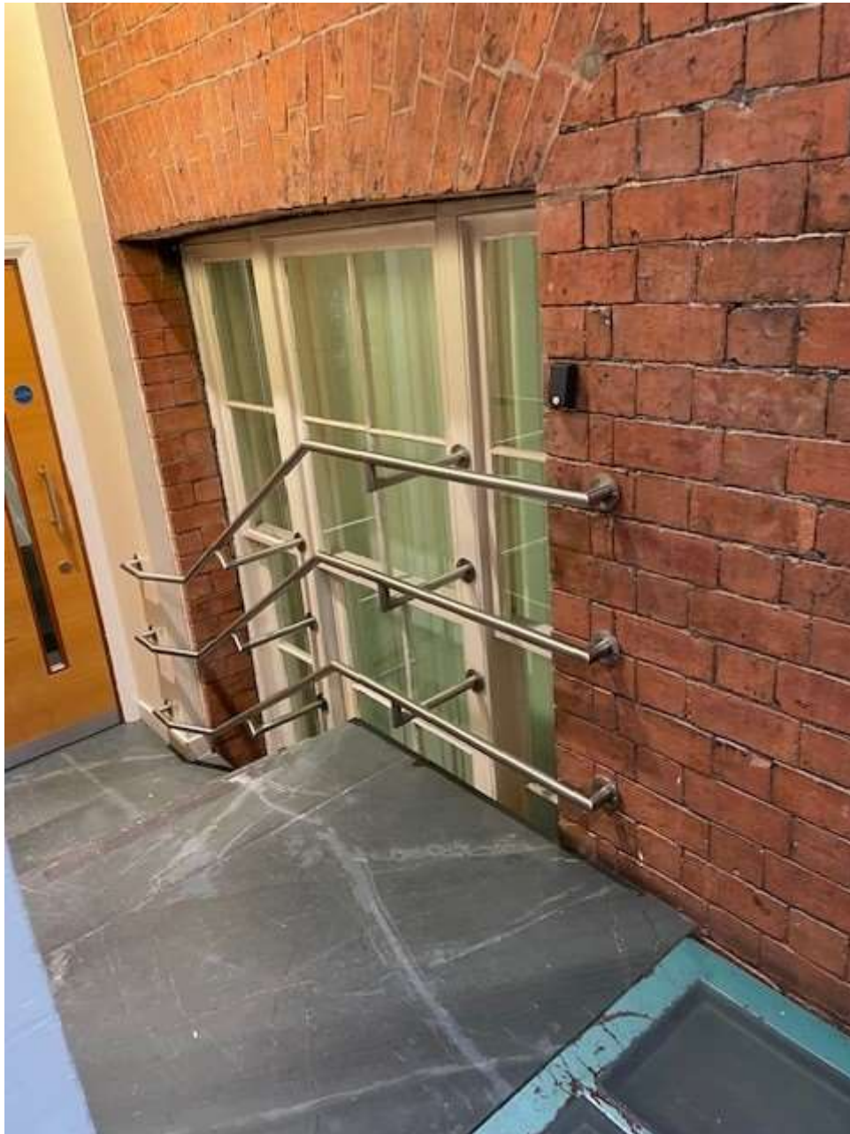
Window 1 (External Before 1995 Refurbishment).
