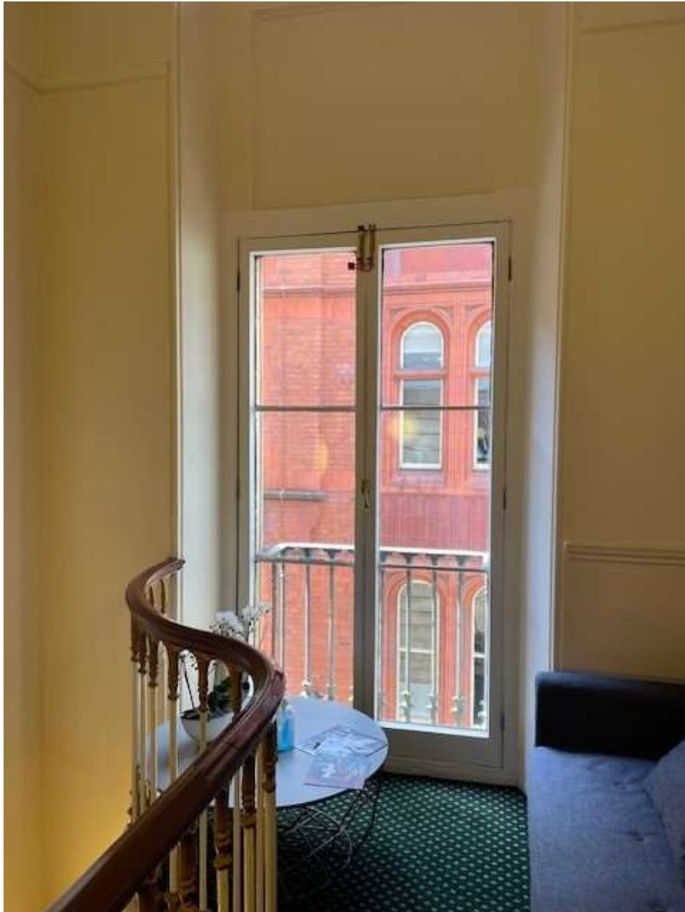
Essex Street Balcony Doors (Internal)
