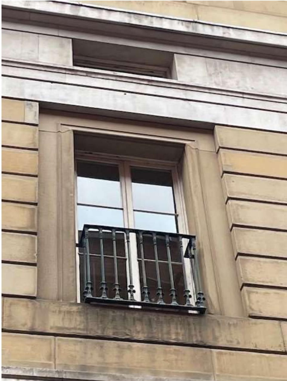
Essex Street Balcony Doors (External)
