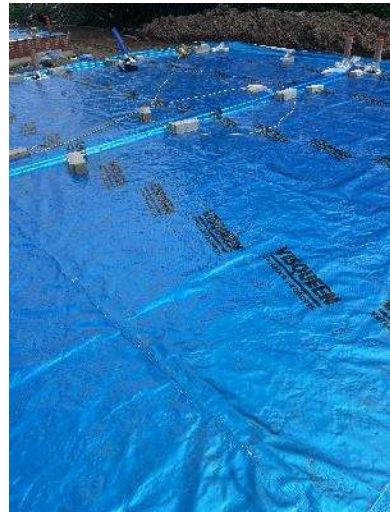
Figure 4 – Membrane in good condition.
