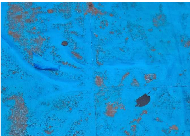
Figure 5 – Hand Welded Seams
