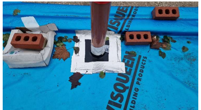
Figure 6 – Service entries sealed and secure.
