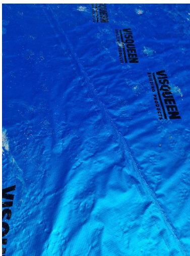
Figure 5 – Hand Welded Seams
