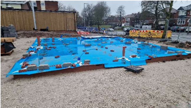
Figure 1 – General view of the plots.
