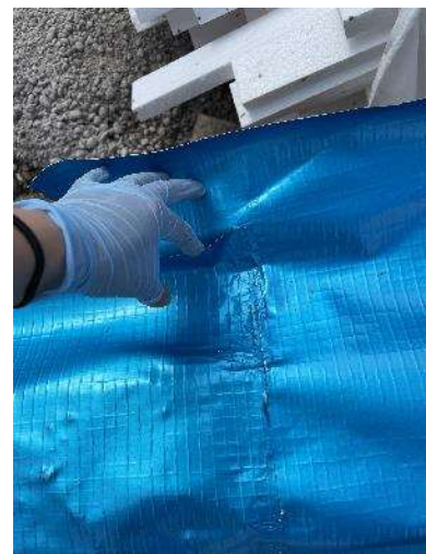
Figure 6 – Joints are hand welded.
