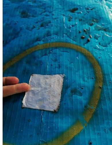
Figure 4 – Gaps in welding have been correctly patched.
