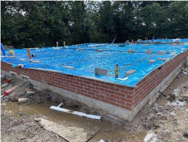
Figure 1 – General view of the plot. Sufficient coverage of cavities.
