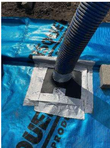
Figure 5 – Service entries sealed on return visit.
