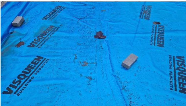
Figure 5 – Hand Welded Seams
