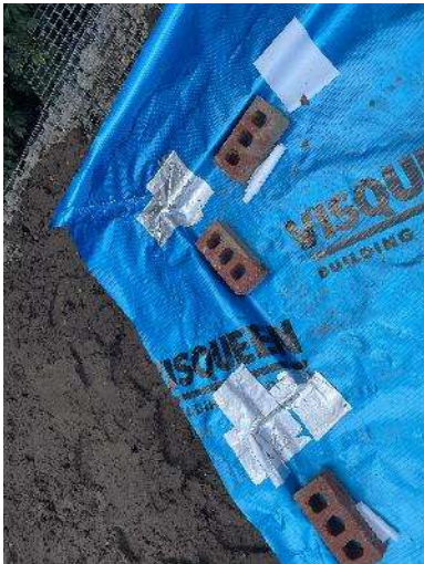
Figure 3 – Corners installed correctly using hand welding and detailing tape.
