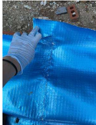
Figure 6 – Joints are correctly hand welded.
