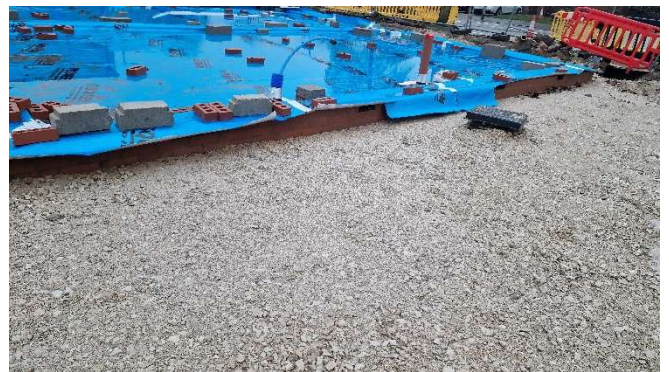
Figure 4 – Sufficient cavity cover.
