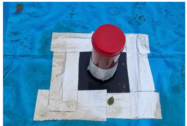
Figure 6 – Service entries sealed and secure.
