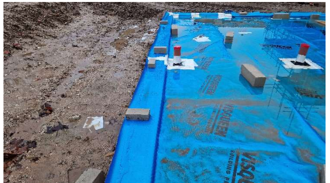
Figure 4 – Sufficient cavity cover, and partial overview
