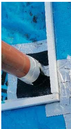
Figure 5 – Gaps in service entry bases correctly sealed.
