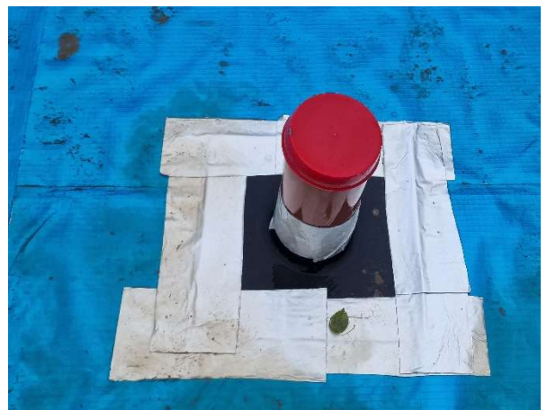
Figure 6 – Service entries sealed and secure.
