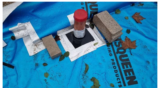
Figure 6 – Service entries sealed and secure.
