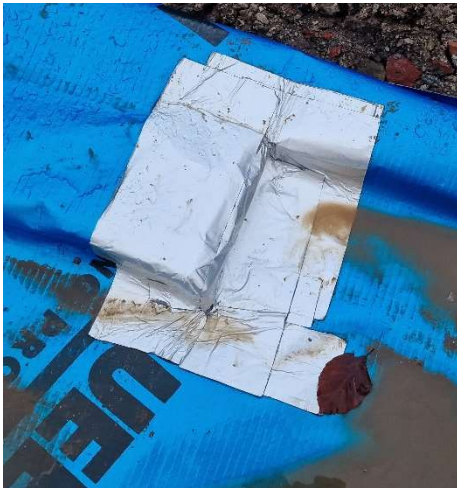
Figure 3 – Corners installed using detailing tape giving sufficient coverage of cavities
