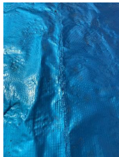
Figure 6 – Joints are hand welded.
