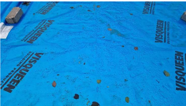
Figure 5 – Hand Welded Seams
