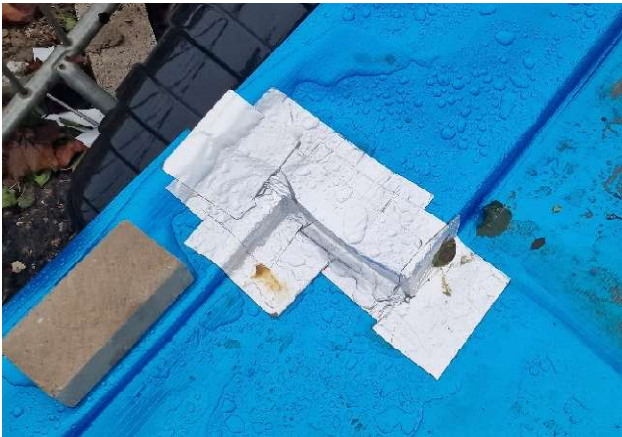
Figure 3 – Corners installed using detailing tape giving sufficient coverage of cavities
