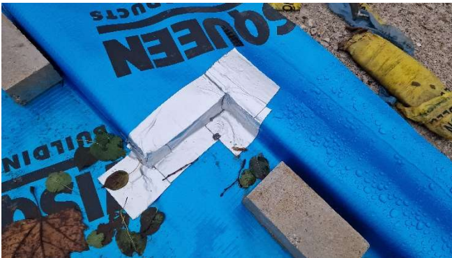
Figure 3 – Corners installed using detailing tape giving sufficient coverage of cavities
