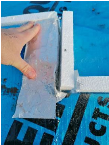
Figure 3 – Gaps in corners correctly patched.
