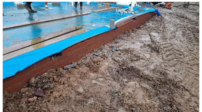
Figure 4 – Sufficient vents, also showing sufficient cavity cover.
