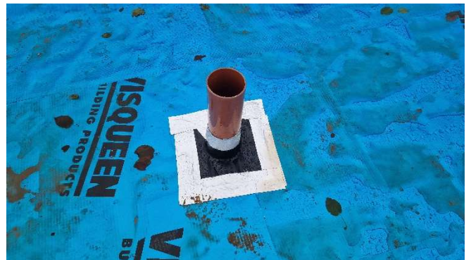
Figure 6 – Service entries sealed and secure.
