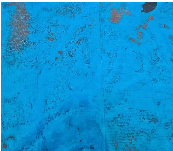
Figure 5 – Hand Welded Seams
