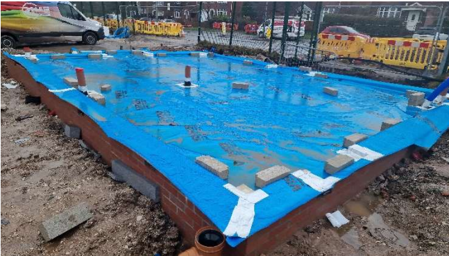
Figure 1 – General view of the plot. Sufficient coverage of cavities.
