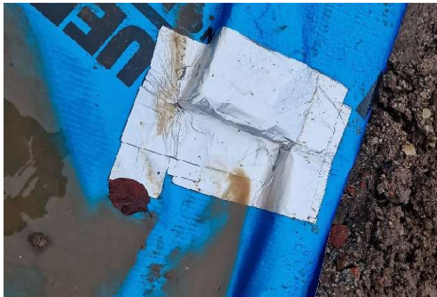
Figure 3 – Corners installed using detailing tape giving sufficient coverage of cavities
