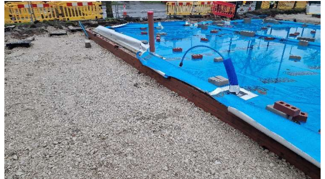
Figure 2 – Sufficient vents. Grill fascia to be installed as brickwork progresses
