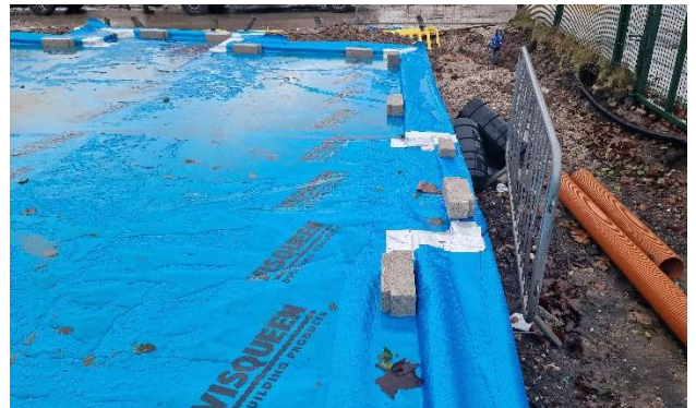
Figure 4 – Sufficient cavity cover.
