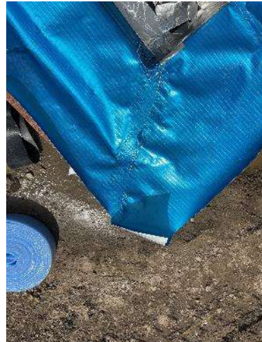
Figure 6 – Joints and corners are hand welded.
