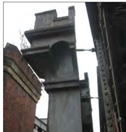
Late steel cables securing free-standing pilaster on its internal face
