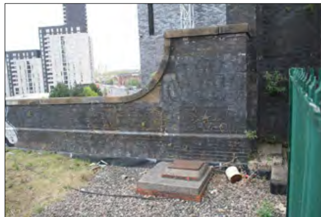
Western approach viaduct: north internal face
