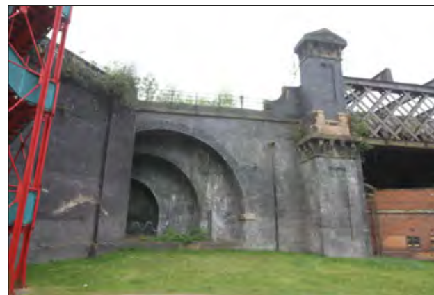
Eastern approach viaduct from the north
