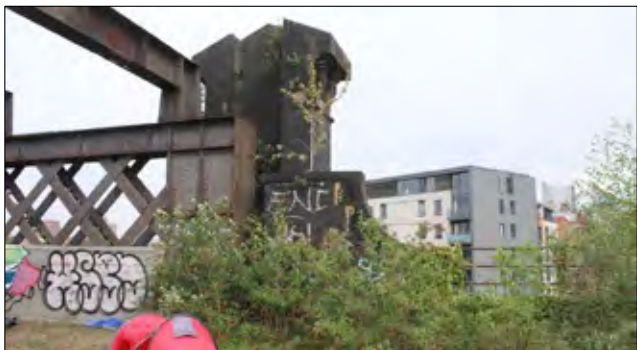
Eastern approach viaduct: north internal face
