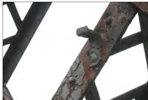
L-shaped bracket rivetted onto the inner face of the north elevation
