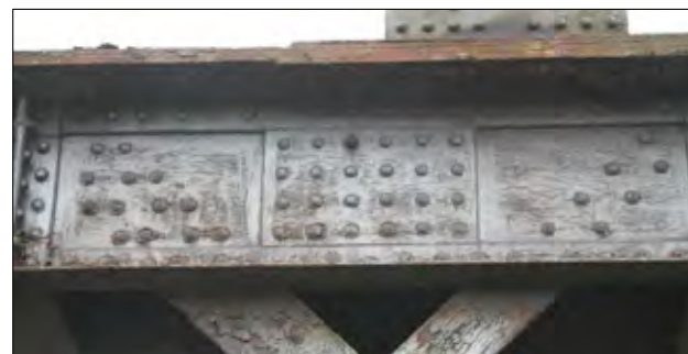
Rectangular jointing plates on the web of the top girder (03a)
