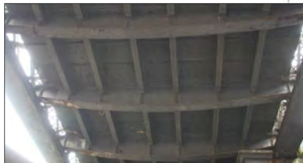
Fish-bellied transverse girders carrying the deck
