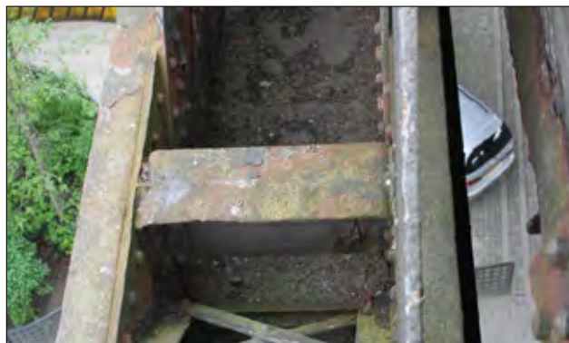
Horizontal T-section bracing bars between webs of bottom girder (03b), forming the upper flange
