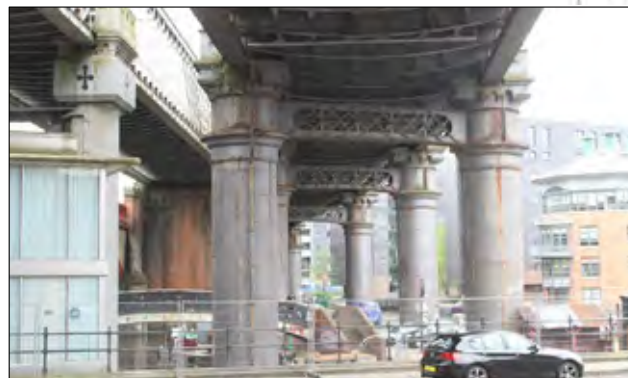
Columns carrying the viaduct
