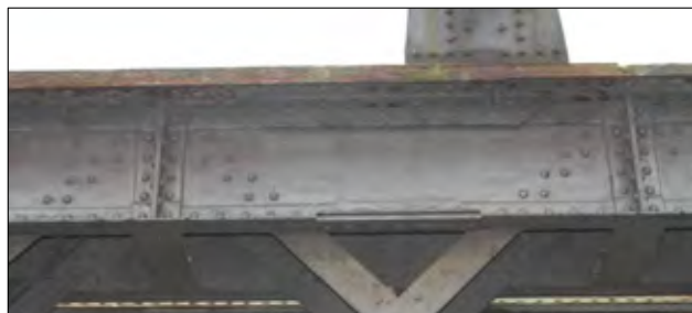
Vertical T-section bracing bars on web of top girder (03a), bolted to horizontal bracing bars forming the lower flange
