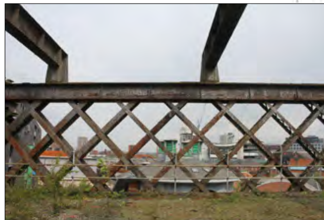
Top girder of the north elevation of the viaduct
