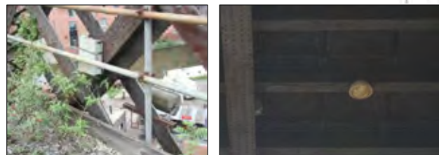
Fuse box and halogen light on the north elevation, with earlier streetlamp attached beneath the deck
