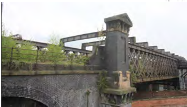
Eastern approach viaduct: detail of decorative pilaster
