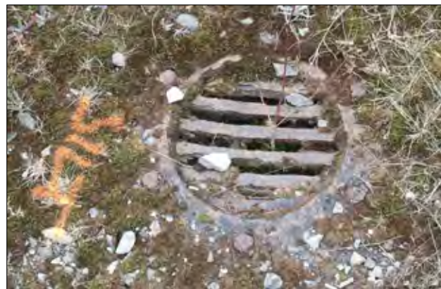
Grate above drainage hopper in deck plate at span joint
