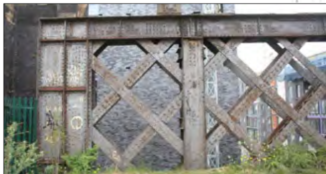
Additional panel at the western end of the north elevation of the viaduct
