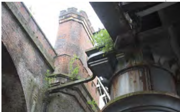
Square-section gutter feeding into downpipe of earlier viaduct to the south
