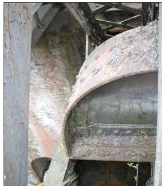
Bull-nosed outer end of fish-bellied transverse girder
