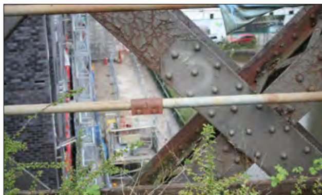
Steel fishplate with chamfered head attached to lattice beam of the north elevation
