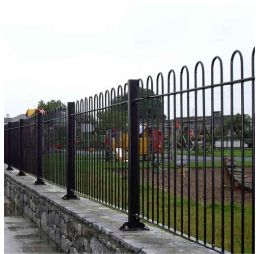
1.2m and 1.8m high brick and looped wrought iron fencing
