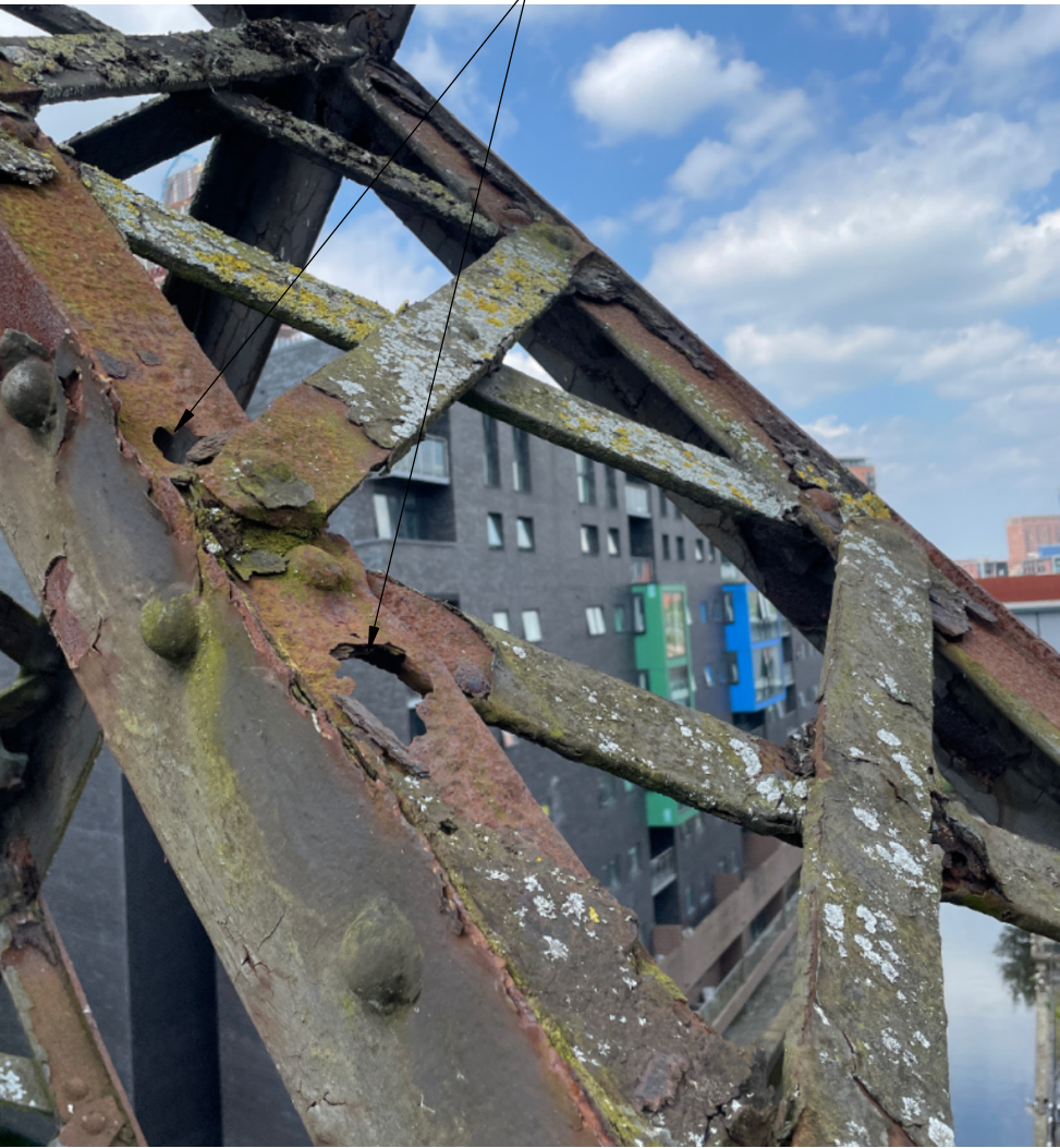
Example 3 - loss of section to inner angle, either side of X-bracing connection - at least 2 holes per length of outstand
