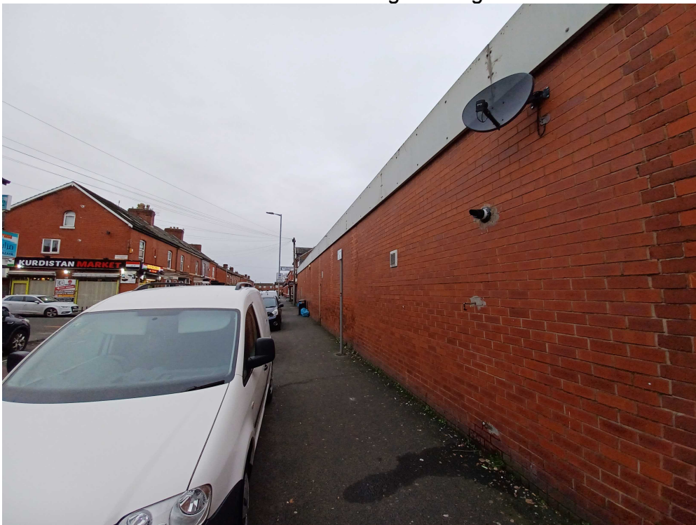
Grandale Road elevation of existing building
