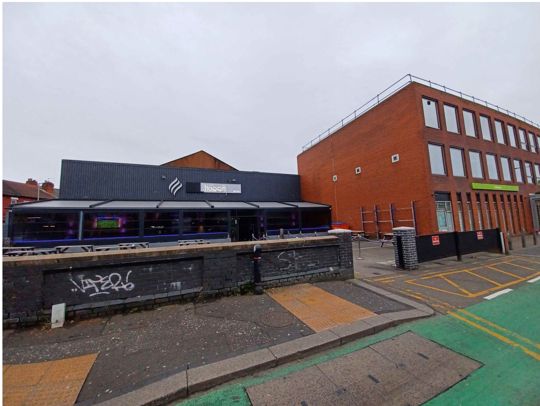
View of adjacent three storey building with the three air vents evident on the gable wall
