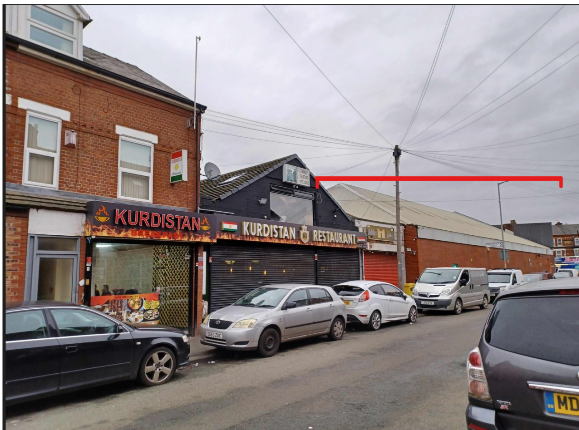
View looking north-east along Grandale Street towards the rear of the application site – the extent of the existing building is highlighted red
