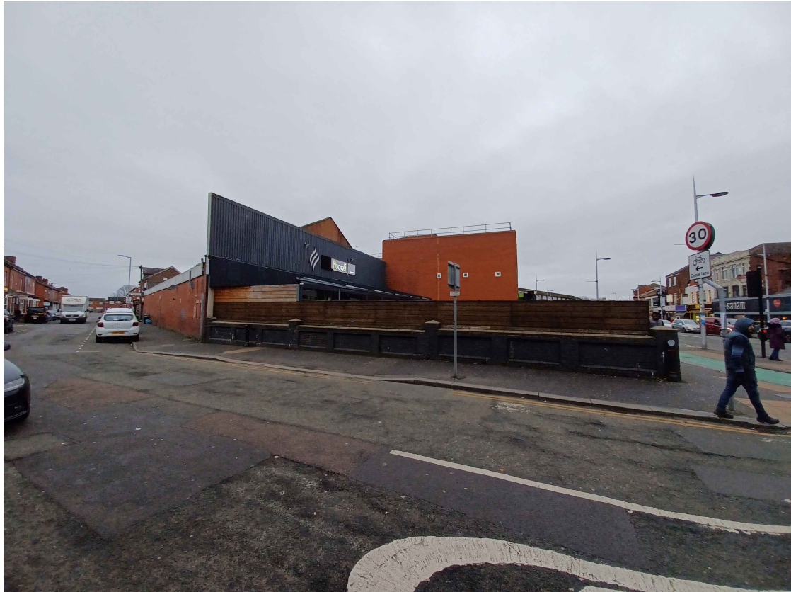
View north across the front of the application site from the corner of Grandale Street and Wilmslow Road, the gable wall of the adjacent building is central to the picture
