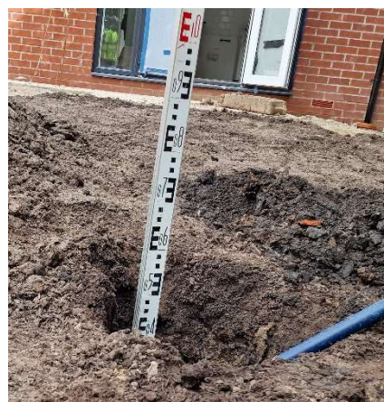
Depth of pit demonstrated at 600mm
