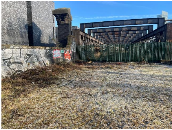
Photograph 12 – Sparsely vegetated land (December 2023)
