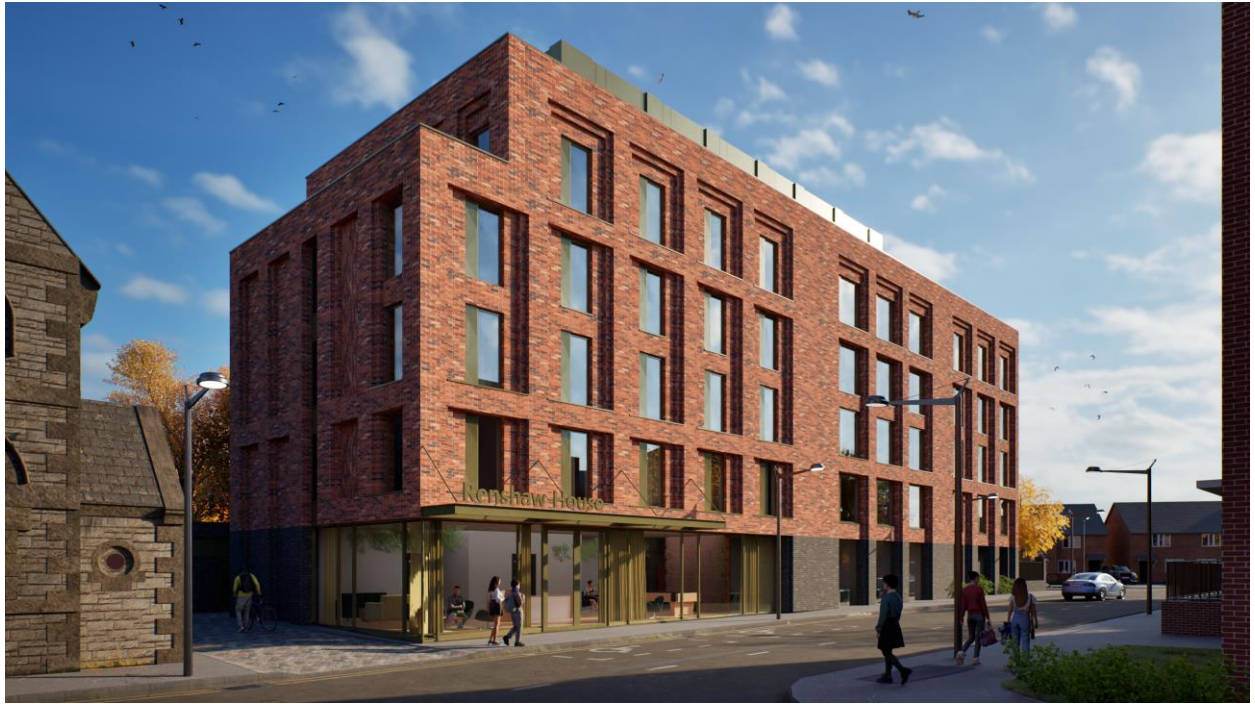
Figure 19: View 1, looking from Hyde Grove into the Site. The former Sunday School building is partially captured to the west of the Site boundary. Source: GWPA Architecture.
