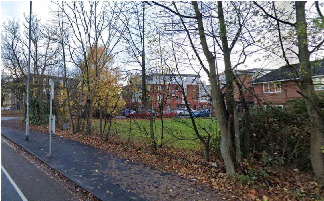
Figure 3: View into the Site and across its tree-lined boundary from Plymouth Grove. Renshaw House is seen to the right of the frame, with other built form on Hyde Grove filtered by the trees. Source: Google Maps.
