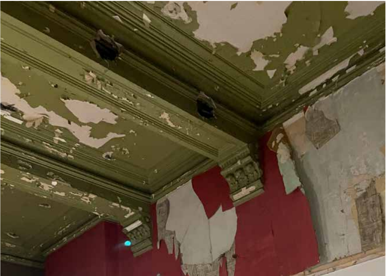
All existing decorative plasterwork will remain exposed- such as these beams and corbels within the ground floor former bank area.
