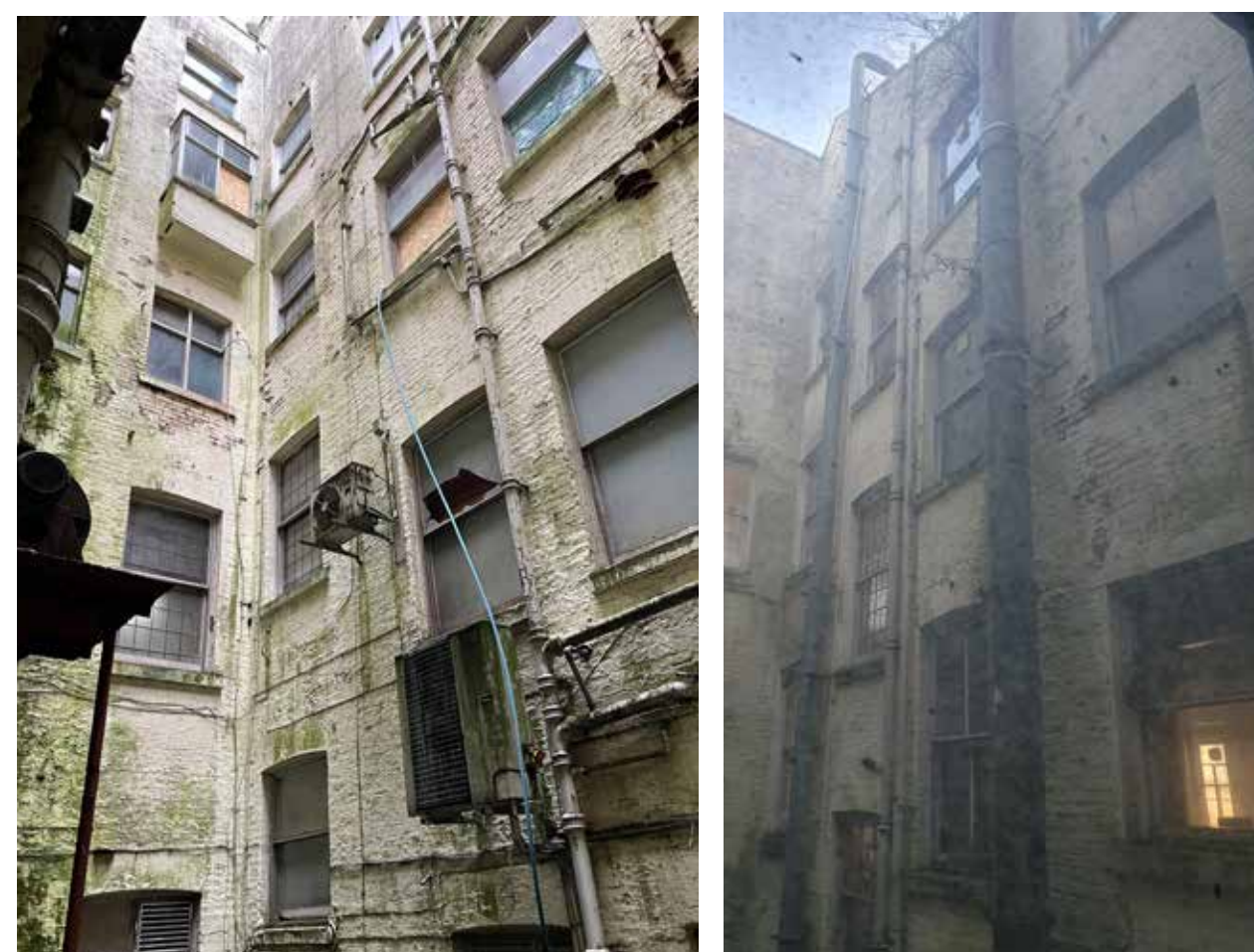
Redundant plant equipment to be removed, and lightwell brickwork cleaned and repaired.
