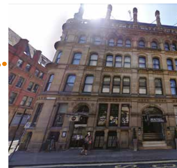
Princess Buildings Grade II Listed
