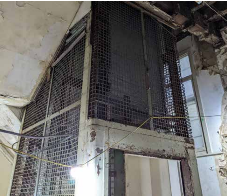
The existing lift will be retained and the enclosure repaired and made safe.
