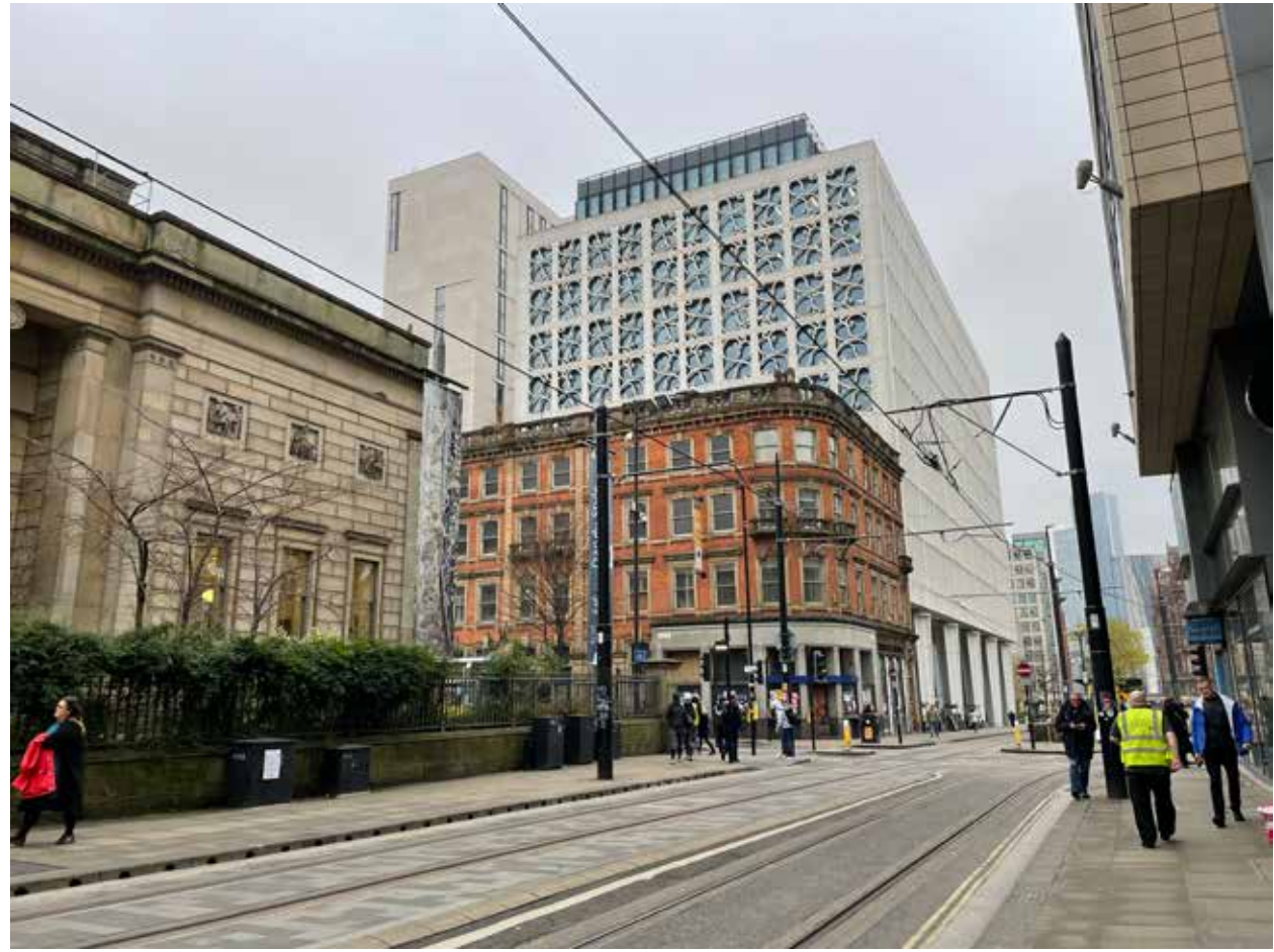
77-79 Mosley Street- Surrounding Context
