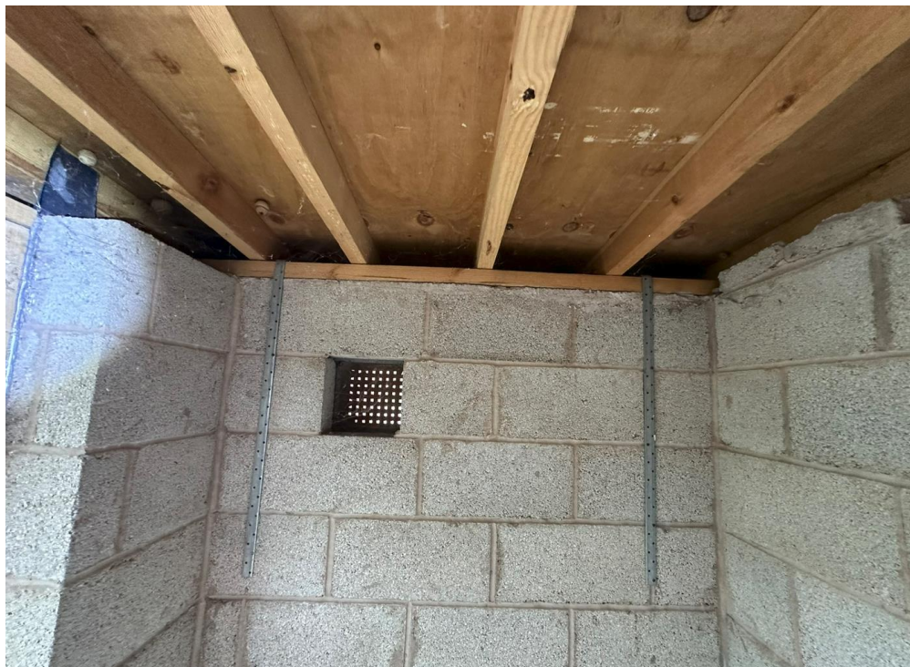
2. Simple Internal roof structure.
