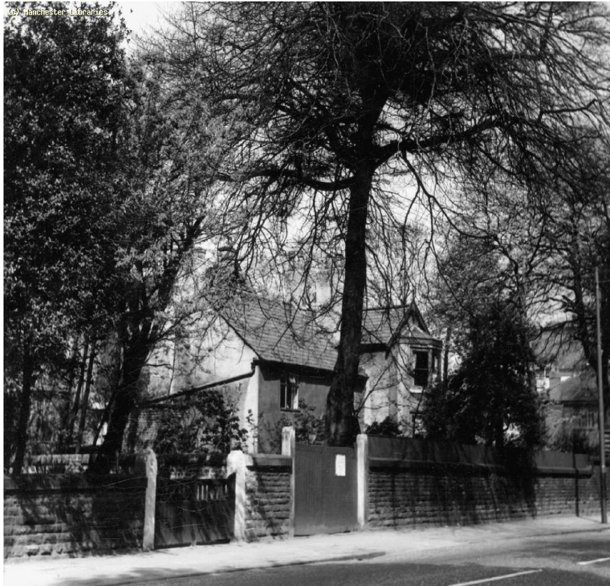
Figure 4.3: 136 and 138 Withington Road (1961)
