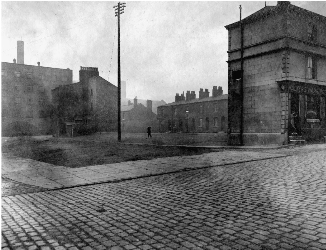
Plate 23: Agnes Street post- partial demolition, 1913, looking southeast.
