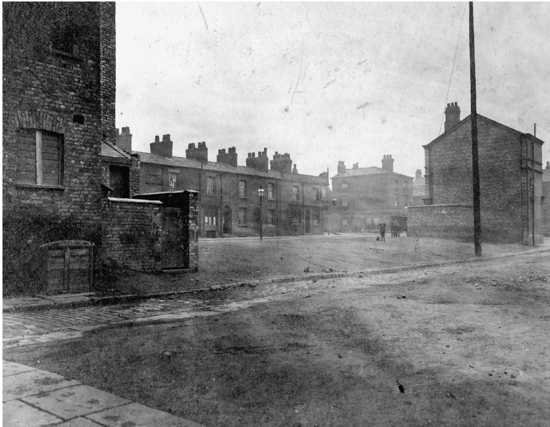
Plate 24: Agnes Street post- partial demolition, 1913, looking southwest.
