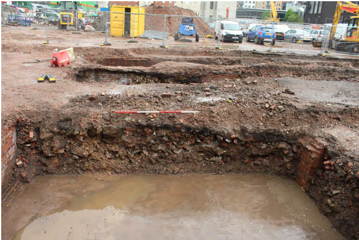
Plate 19: Factory basement G9 demolition backfill, looking southwest, 2m scale.
