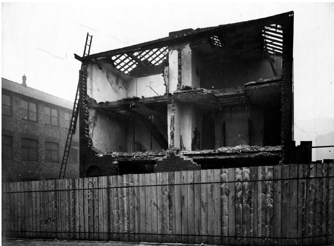
Plate 26: Newcastle Street demolition, 1908.
