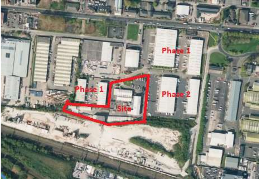
Figure 6 - Development phasing - areas marked Phase 1 and Phase 2 were re-worked to a depth of approximately 5 metres.
