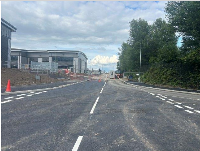
Pictures 8 shows the private road into the site at the side arm junctions.
