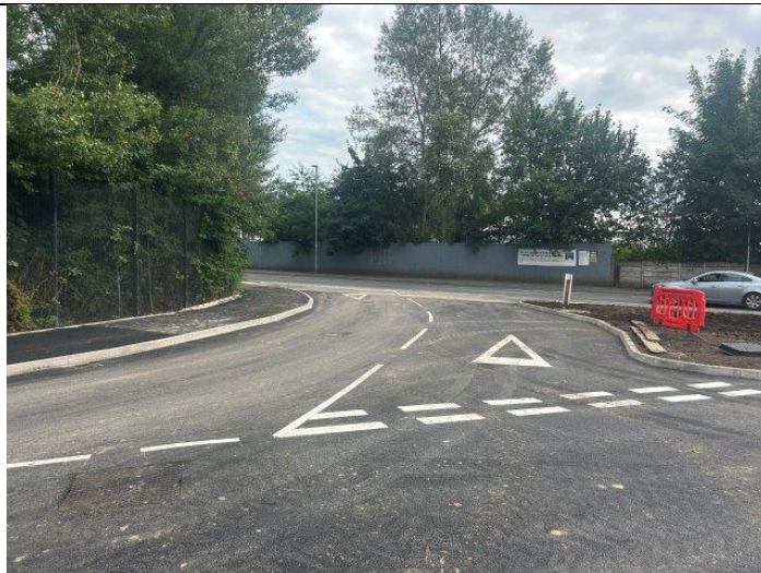
Pictures 2 shows the southern access arm road markings.
