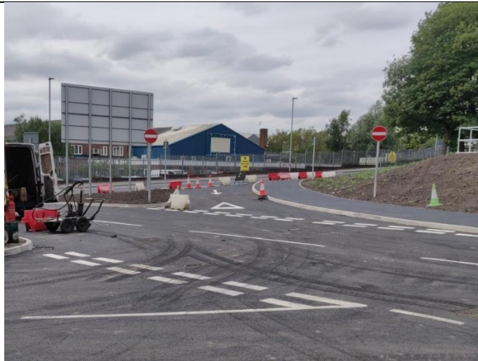
Pictures 7 shows the Northern access arm road marking and signage.
