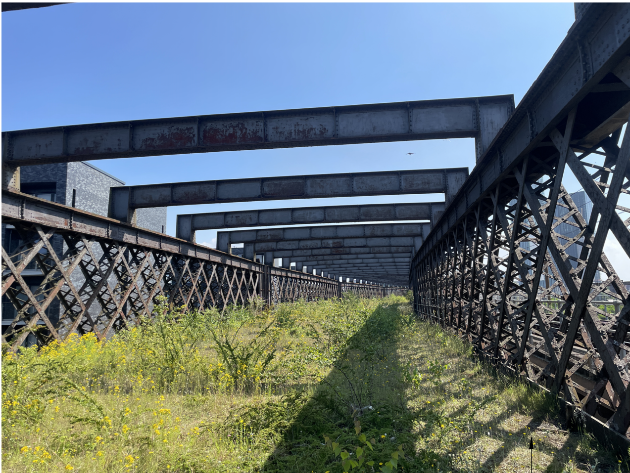
Typical existing ballast and vegetation to Ph2 steel spans
