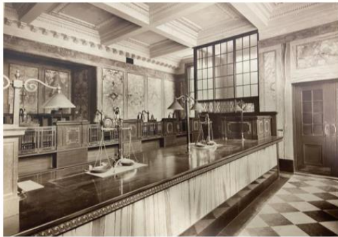
Original image of the ground floor Banking Hall interior
