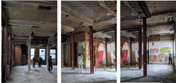
Recent interior views of the Banking Hall, showing condition following soft strip out works
