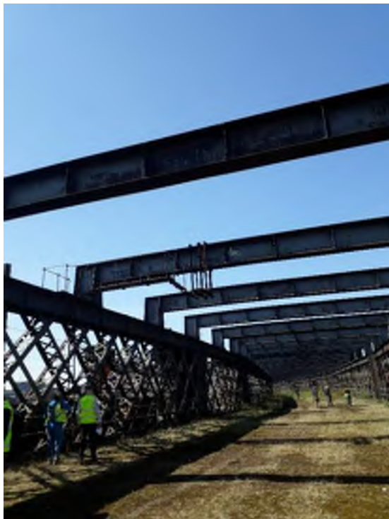
Plate 11: Metals structure attached to southern overhead girder.
