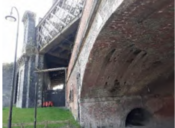
Plate 2: Red brick arches supporting the railway line below the viaduct (looking towards northern boundary).
