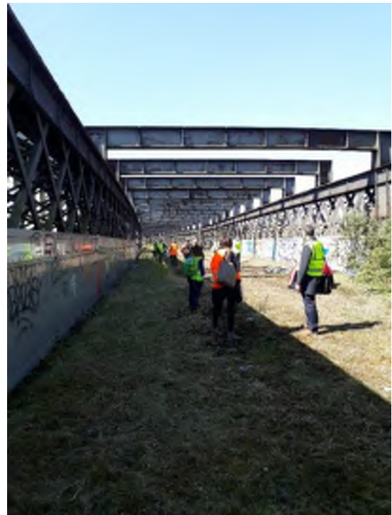
Plate 8: Eastern area of viaduct looking west. Barrier on northern and southern side of viaduct in this locality which prevents debris falling to the railway line below.
