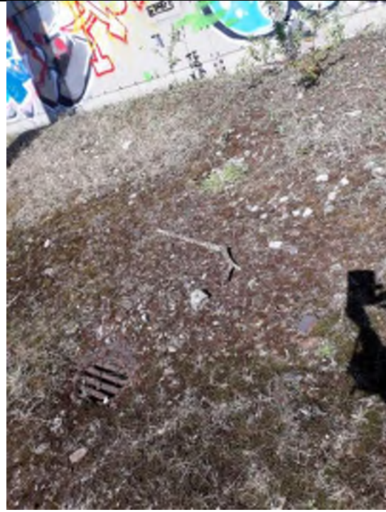
Plate 10: Drainage grid visible on surface of viaduct.
