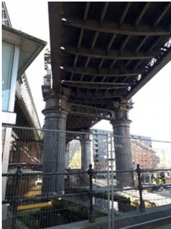
Plate 3: Underside of central/eastern area of the viaduct looking west over Bridgewater Canal basin. Footbridge over canal is shown on the left side of photograph.
