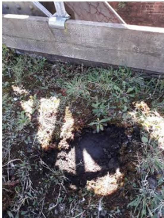
Plate 12: Variable thickness of ballast with base of viaduct visible in some locations.
