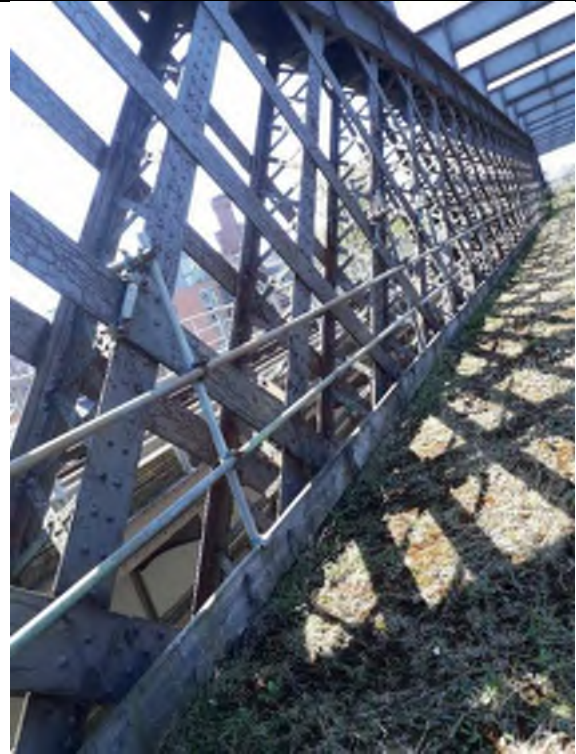
Plate 22: Scaffolding and kickboard along areas of viaduct. Looking south to tramline to south of site.
