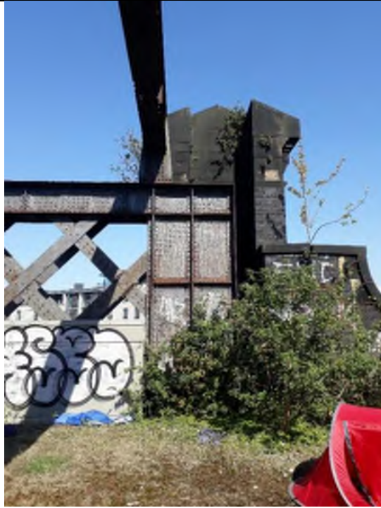
Plate 9: Tent and sleeping bag in eastern area of viaduct.
