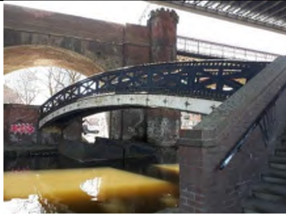
Plate 5: Foot bridge over part of the Bridgewater Canal in central/eastern area below viaduct.
