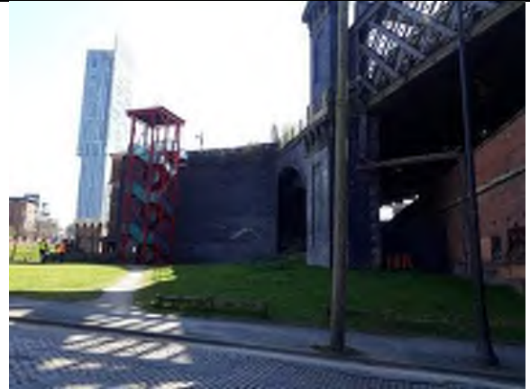
Plate 6: Grassed area to north of viaduct along eastern length of viaduct. Staircase shown in left of photograph which provides access from ground level to car park above and viaduct.
