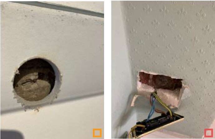
Example of modern lining and wallpaper covered plaster from investigation works. Refer to investigation works document for further photos.
