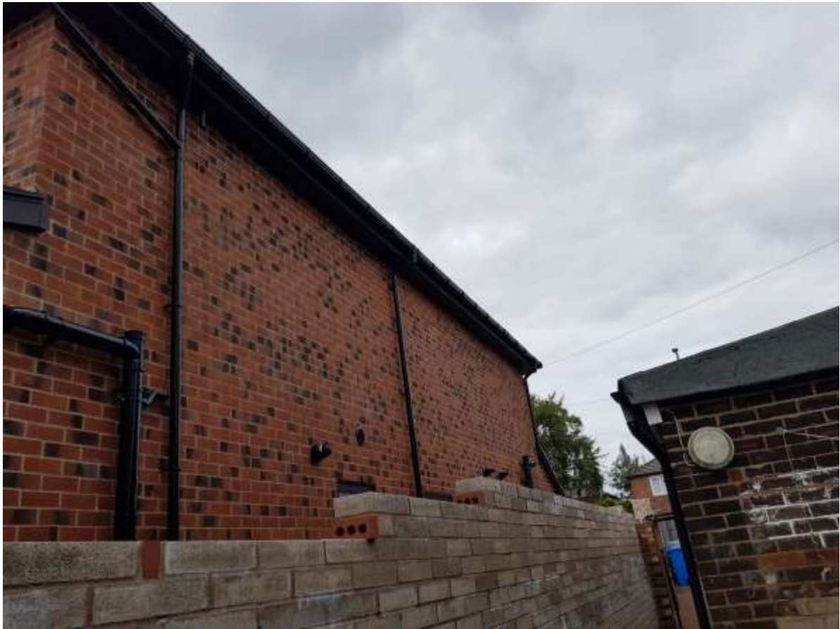
Gable wall of No.142 Nuthurst Road – no main room windows
