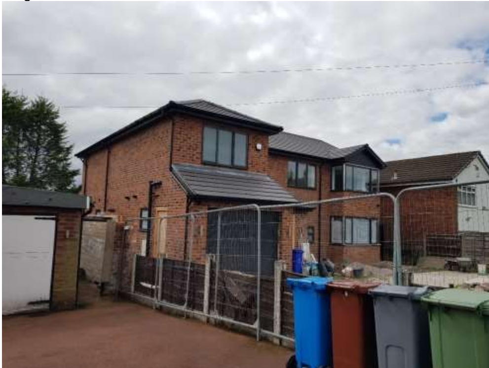
Neighbour at No.142 Nuthurst Road front elevation
