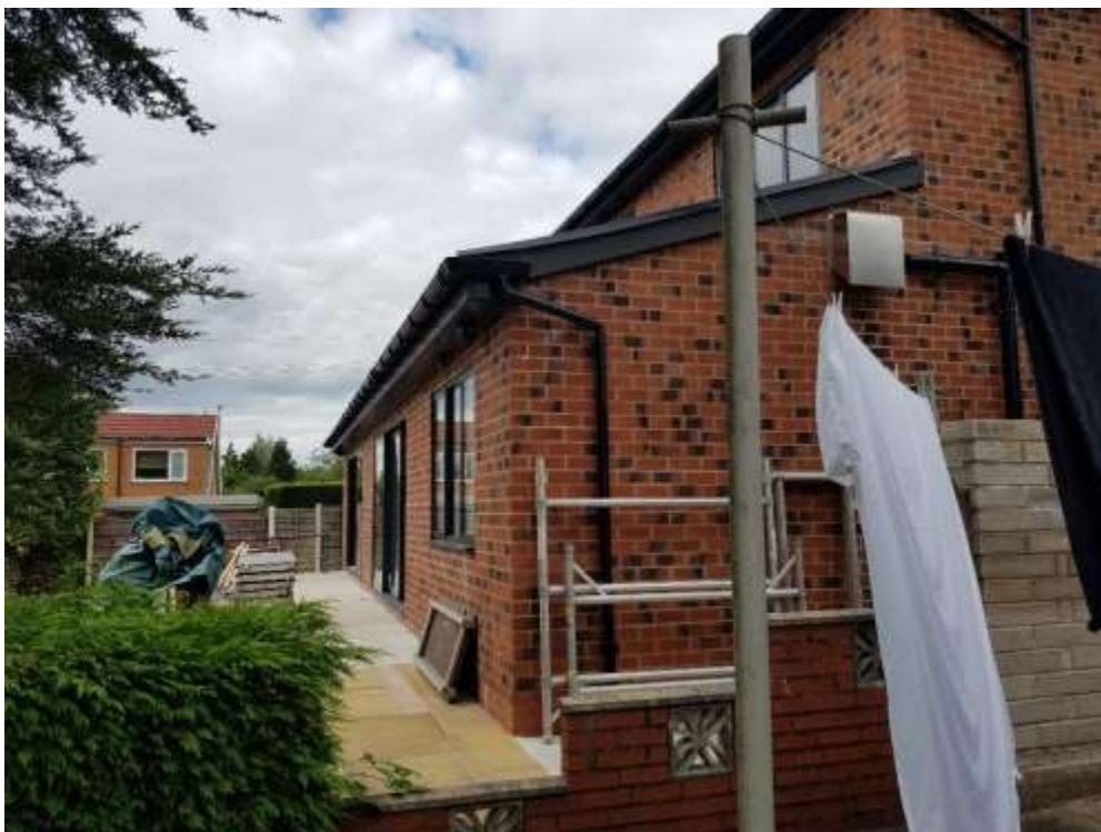
Neighbour at No.142 Nuthurst Road full width rear extension
