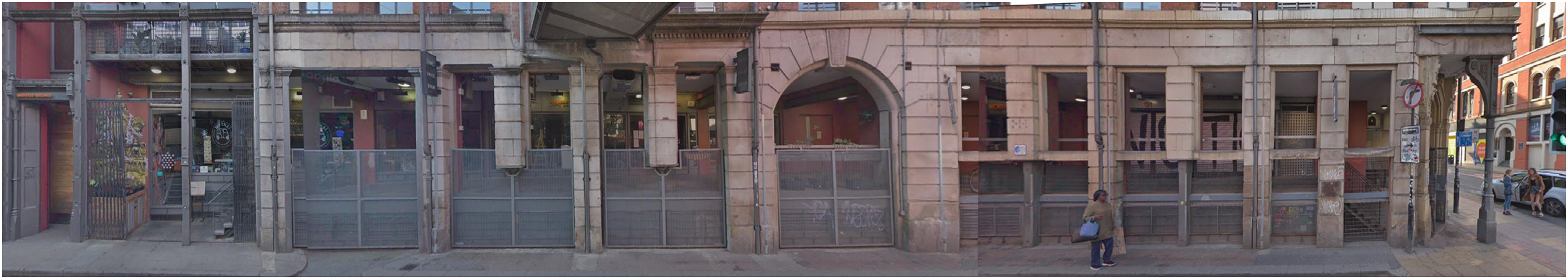
PHOTOGRAPH OF THE EXISTING TIB STREET FACADE
