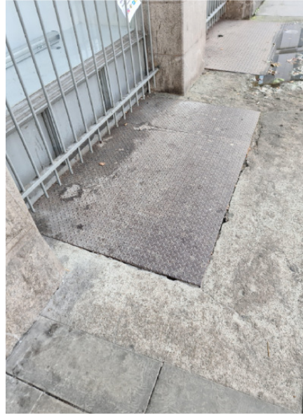
Photo of existing metal plate
