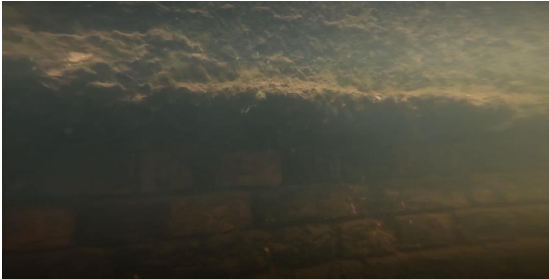
Photo 46: General underwater view of brickwork and concrete plinth below water level at chainage 44m.
