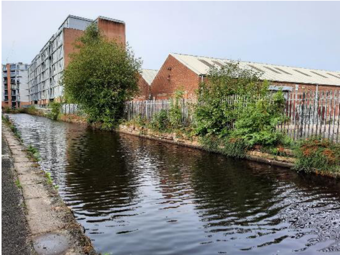
Photo 3: View looking LH at chainage 60m
