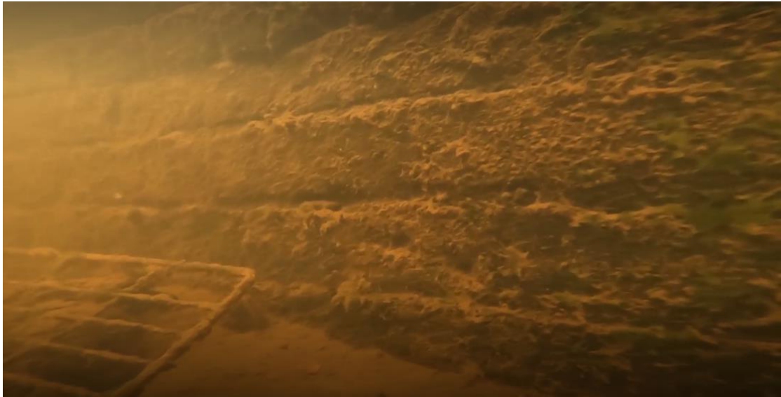
Photo 48: General underwater view of stonework and debris to invert at chainage 150m.
