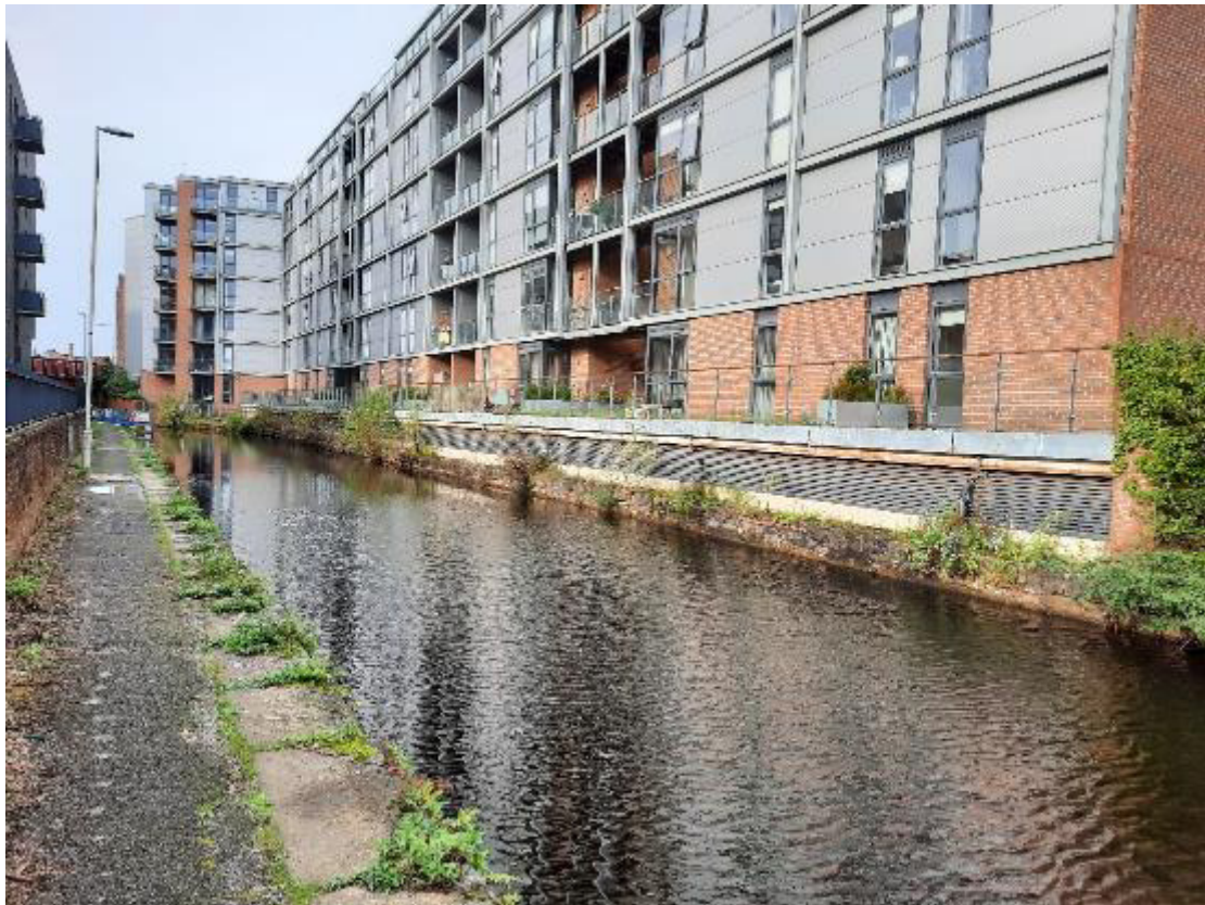
Photo 1: View looking LH at chainage 0m
