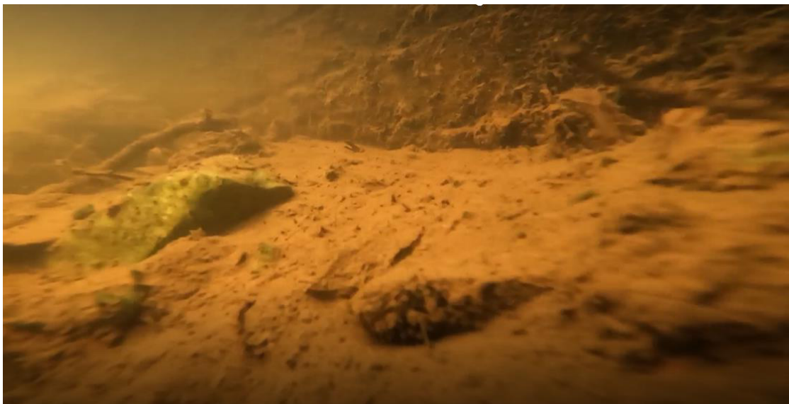
Photo 47: General underwater view of invert at chainage 148m.
