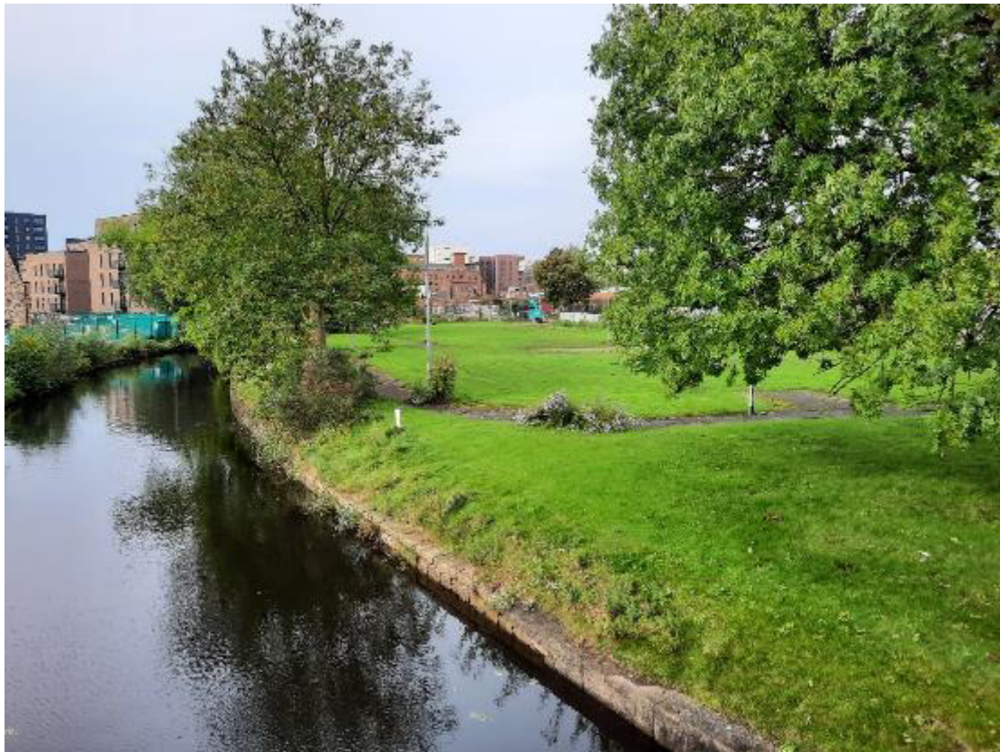
Photo 9: View looking LH at chainage 238.5m
