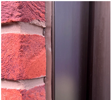
Mastic as built on VMU
