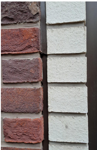
Proposed mastic installation (bottom section)
