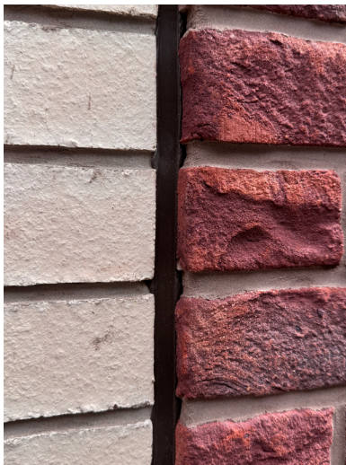
Mastic spilling
