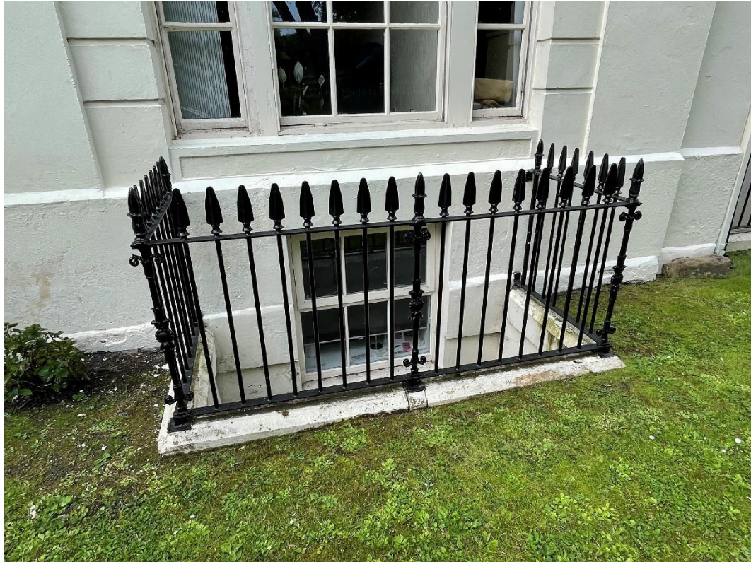
Figure 4.7: Detail of basement light well
