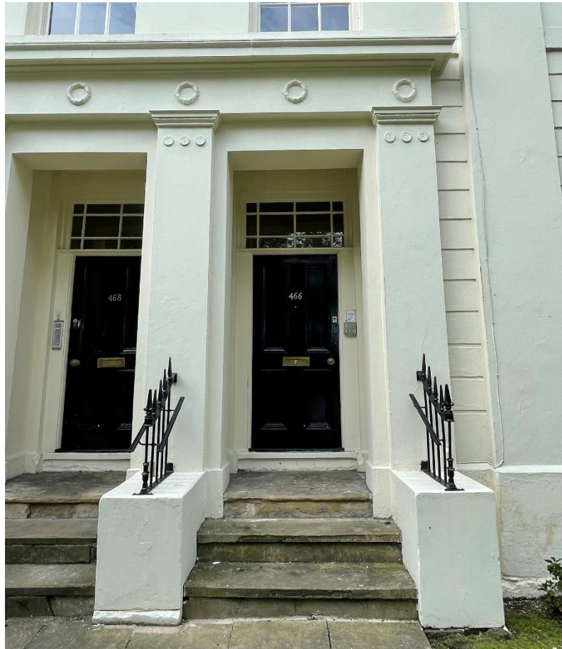
Figure 4.2: Detail of entrance doorway to 466
