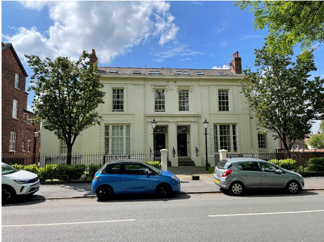
Figure 4.9: View of 466 and 468 from the opposing side of Moss Lane East
