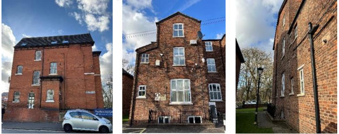
Figure 4.12: East facing, rear facing and west facing elevations of 470 and 472 Moss Lane East
