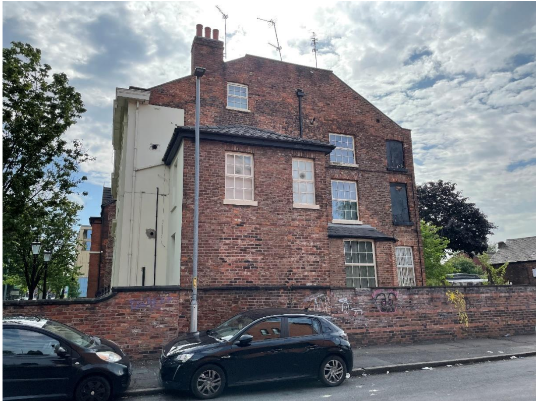
Figure 4.3: West facing elevation of 466 and 468 Moss Lane East
