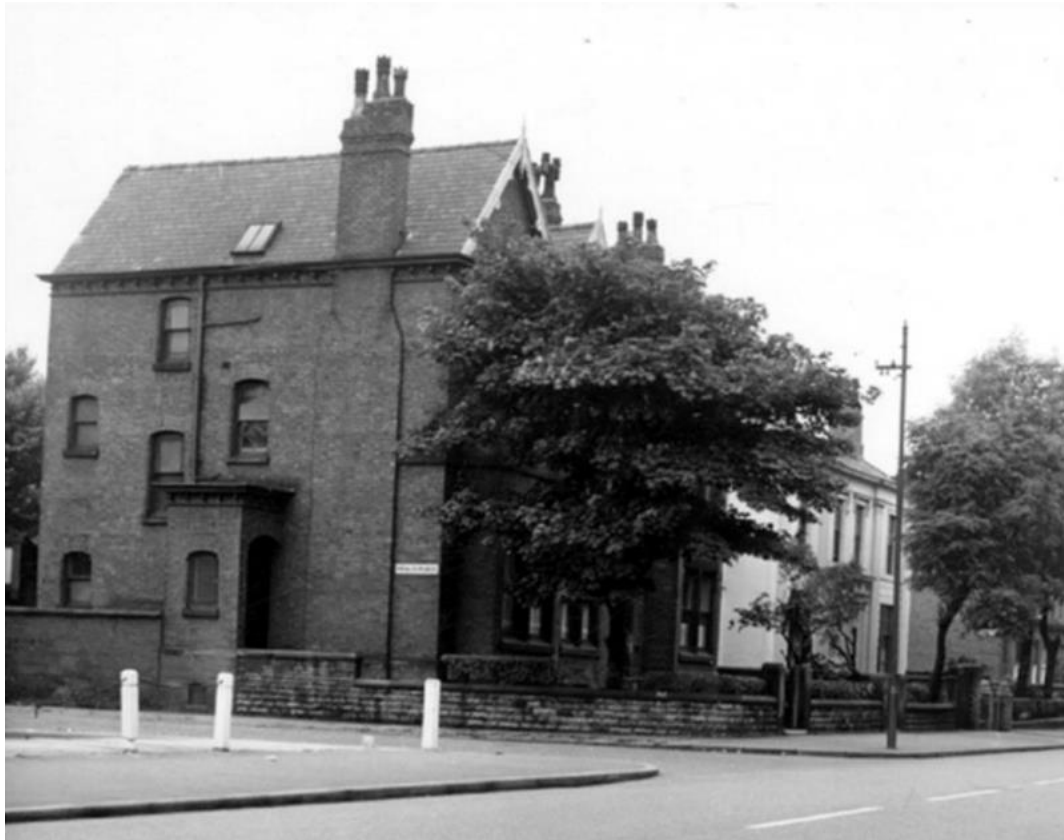
Figure 4.13: East facing elevation of 470 to 472 Moss Lane East in 1969 (Source Manchester Image Library)
