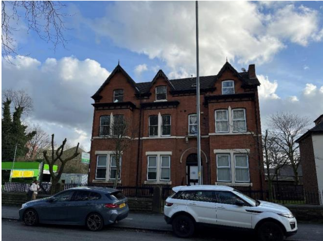
Figure 4.11: North facing elevation of 470 to 472 Moss Lane East
