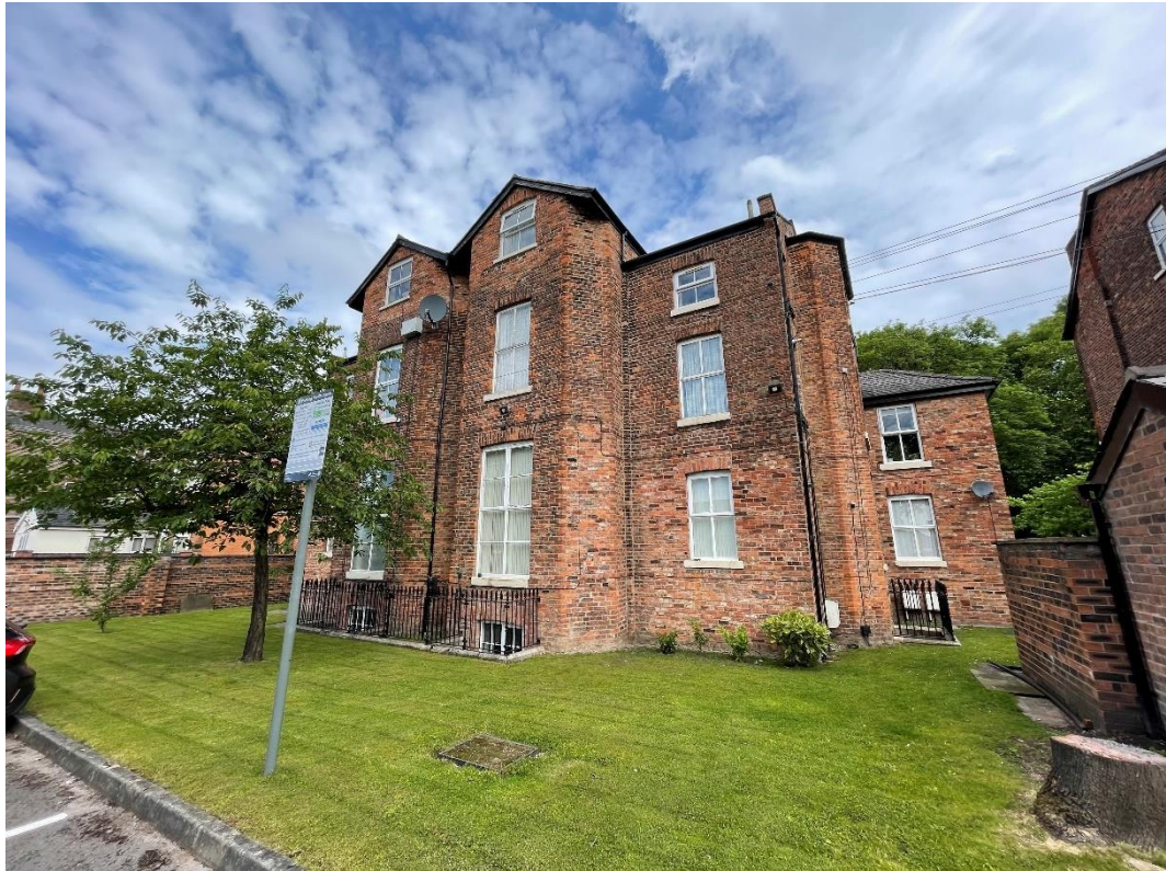
Figure 4.4: Rear facing elevation of 466 and 468 Moss Lane East
