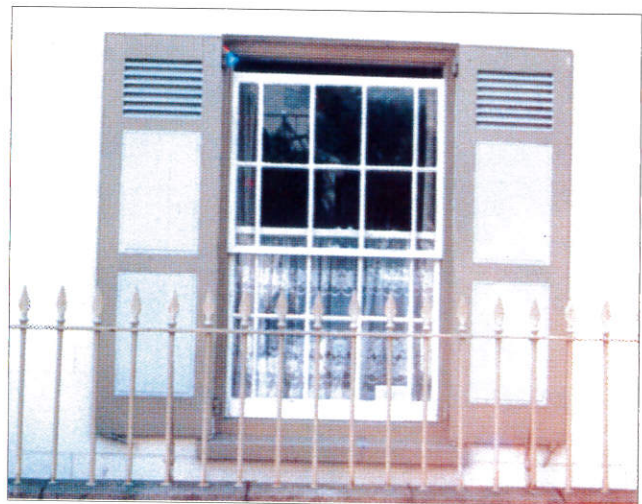
Two types of shutter found in St Helier - a louvred shutter with "keyhole" detail and a solid shutter. Note how the colours have been picked out to match the sash window boxes, cills and railings.
