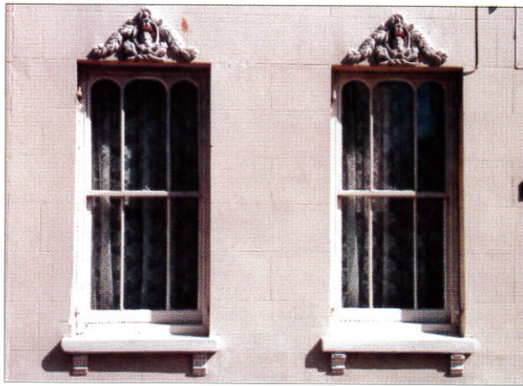
A pair of pretty sash windows with curved upper sashes and render detail above, St Helier
