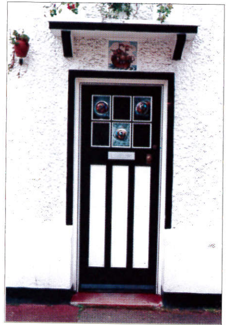
Typical 1930s door with three vertical panels, St Helier
