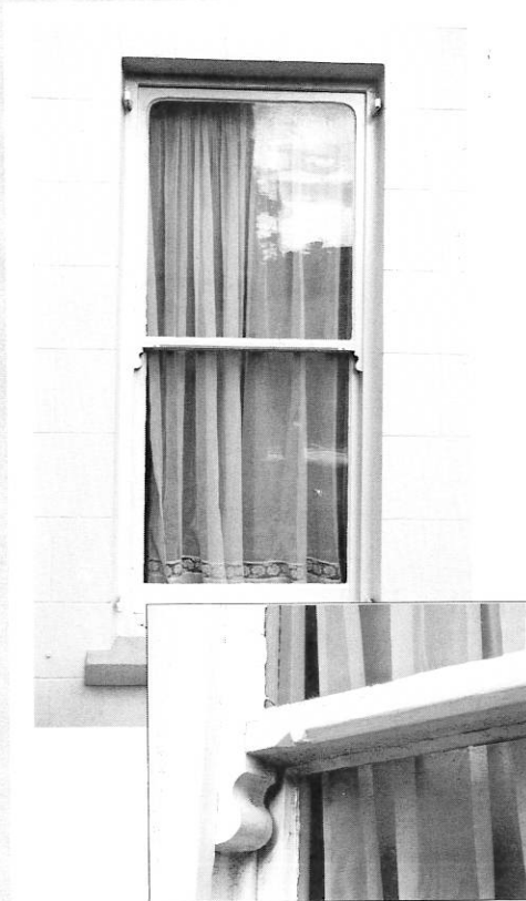
Single-pane sash with chamfered meeting rail, diamond chamfer stop and decorative horns, St Helier
