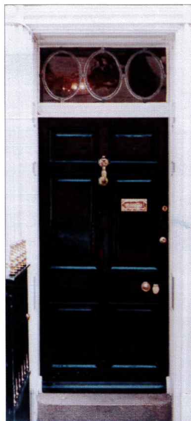
Six raised-and-fielded panel door, with fanlight over, St Helier
