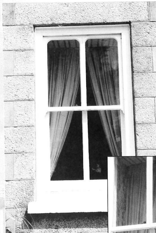
Four-pane sash with grooved central vertical glazing bar and an alternative style of horn, St Martin
