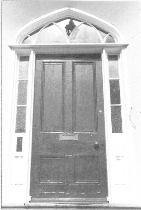
Four-panel door with side-lights and arched Gothic fanlight, St Saviour
