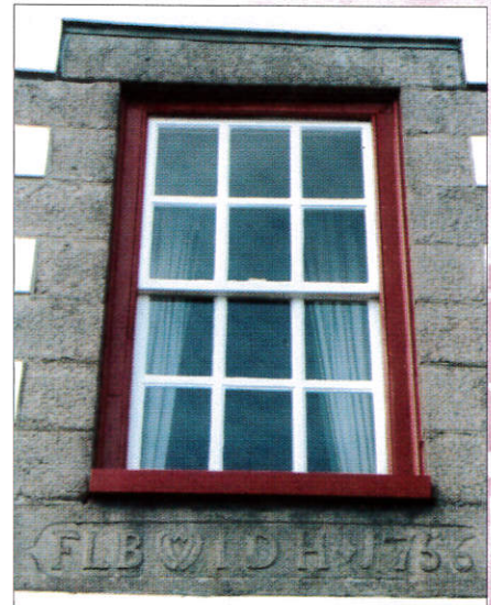
One of the earliest sash windows in St Helier at Hue Street - the building is dated 1756. Note the very wide & flat glazing bars, typical of this early style.
