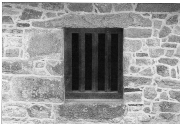
Chamfered timber mullions, designed to allow the infiltration of as much light as possible, Hamptonne, St Lawrence.
