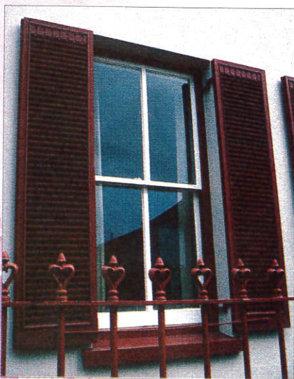
Two types of shutter found in St Helier - a louvred shutter with "keyhole" detail and a solid shutter. Note how the colours have been picked out to match the sash window boxes, cills and railings.
