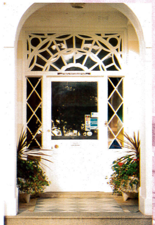
Half glazed door with large elaborate fanlight extending across glazed sidelights, St Brelade
