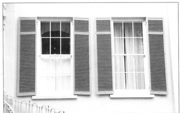
A fine pair of traditional 12-pane Georgian sash windows, complete with external and internal shutters, St Helier
