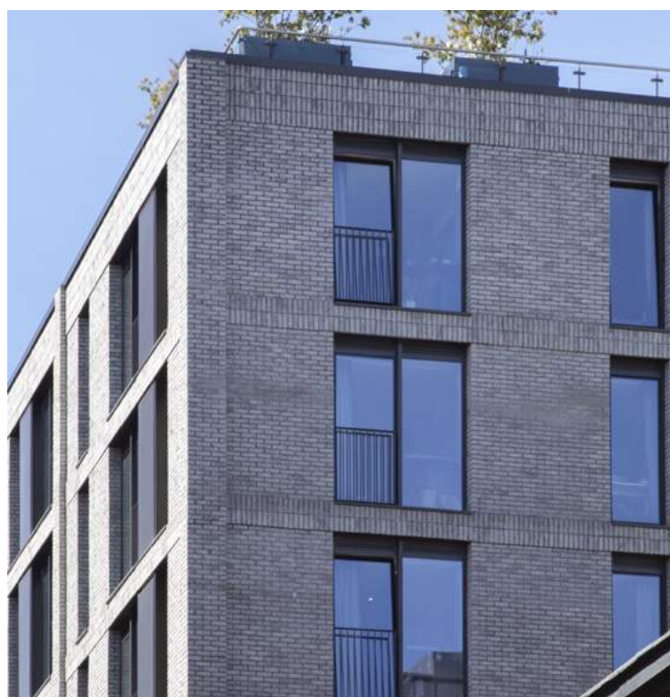
Using a single brick type, brick detailing is used to emphasise an area
