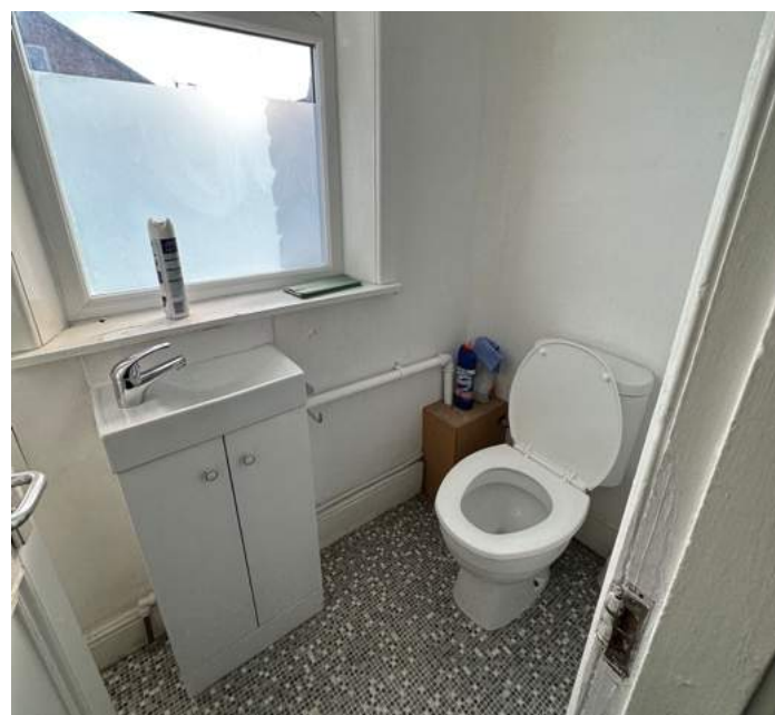
One of the WC windows to be blocked up and ventilation installed
