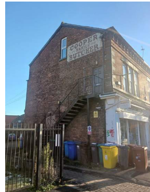
The Passageway Access to the Side of The Site
