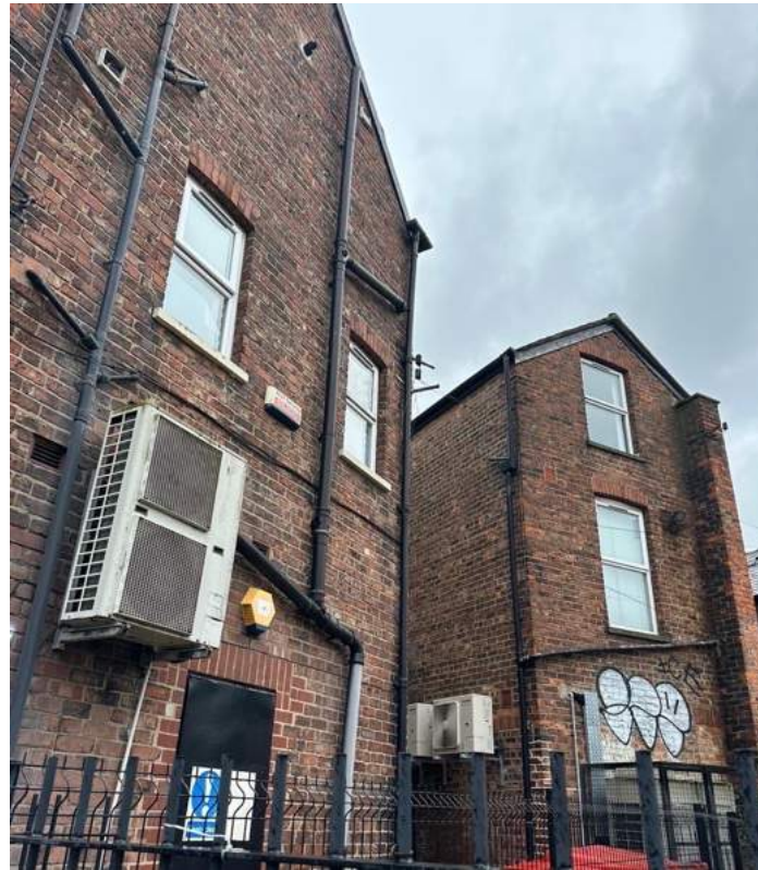
Windows to the rear of the adjacent building at first and second floor
