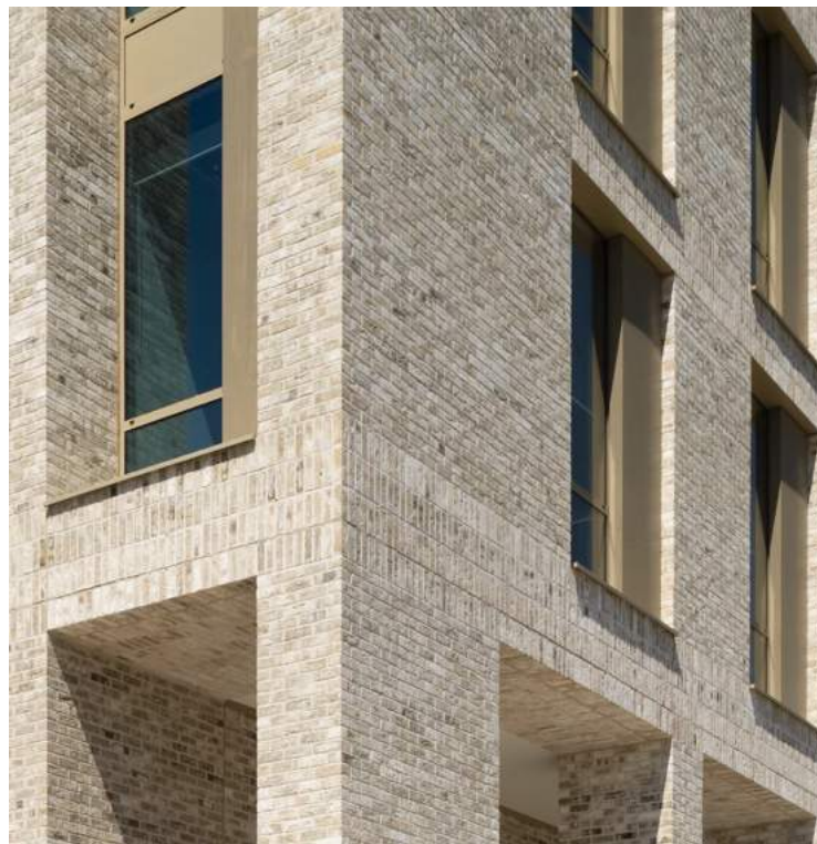
Brickwork detailing to create varying of texture compared to areas of plain brickwork using the same brick throughout
