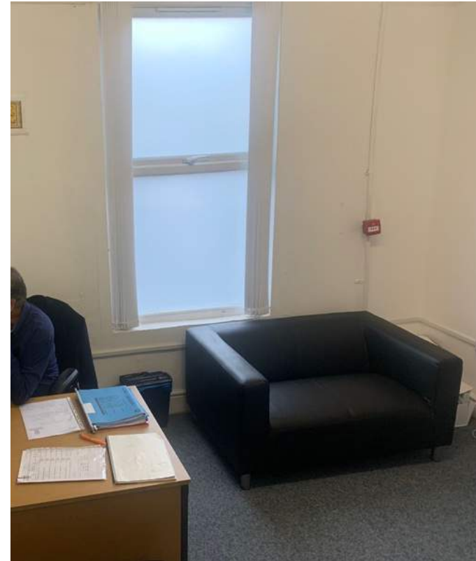
First Floor Office Window to be relocated
