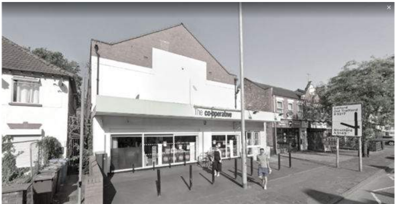
Existing building- Demolished 2023-2024
