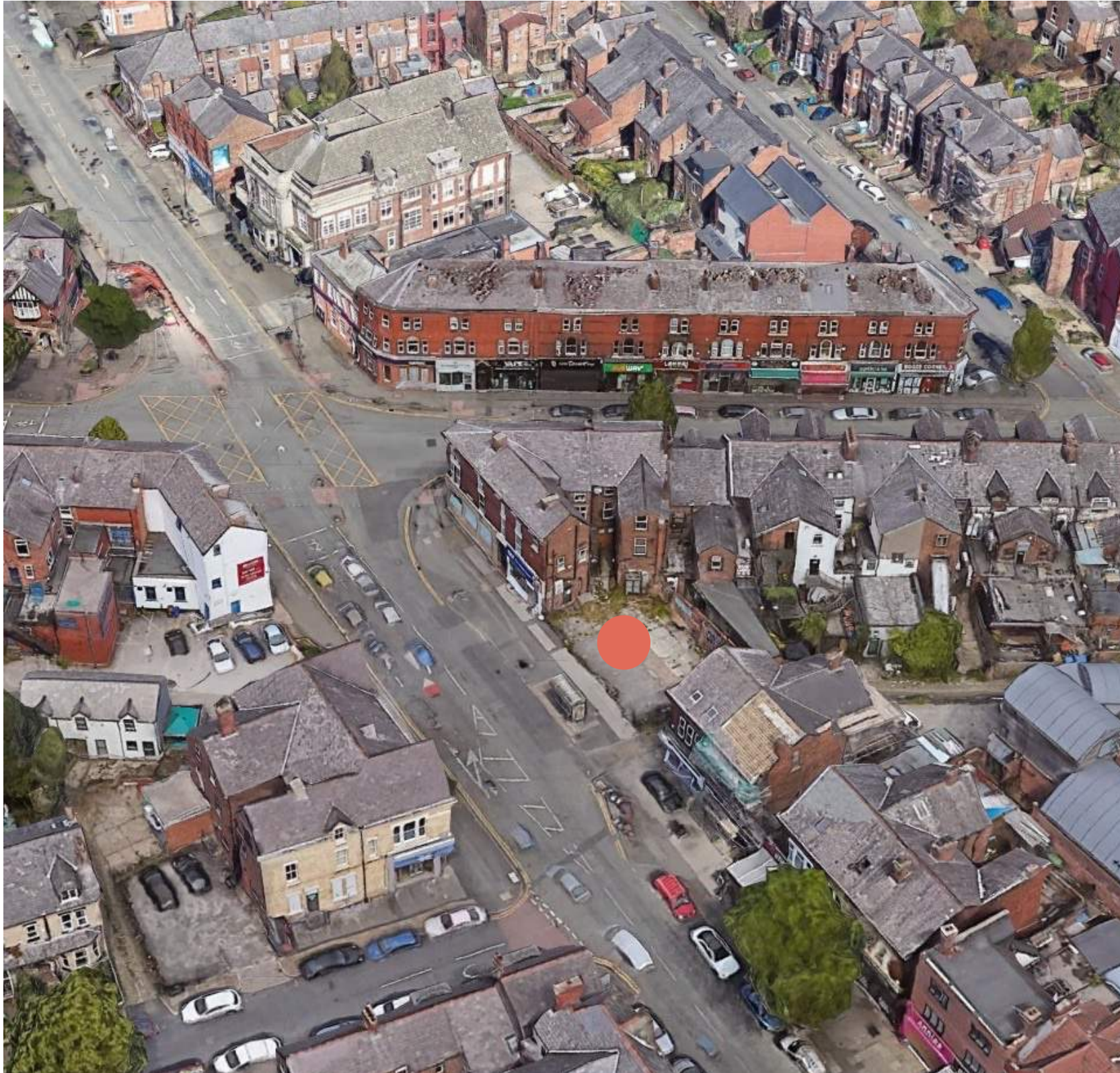
Aerial view of the Main Junction between Wilbraham Road and Barlow Moor Road
