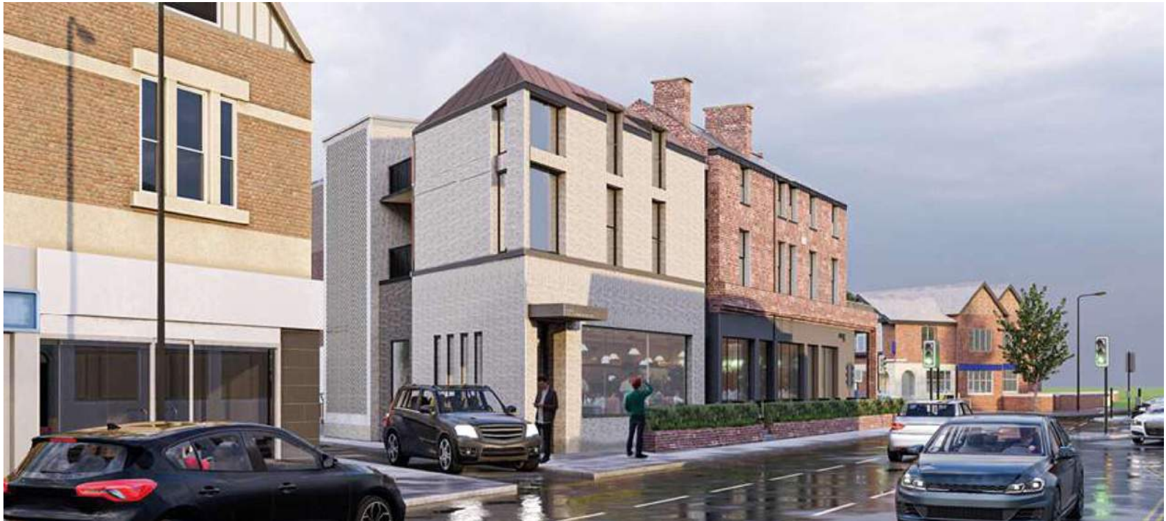
Kemps Corner viewed from Barlow Moor Road
