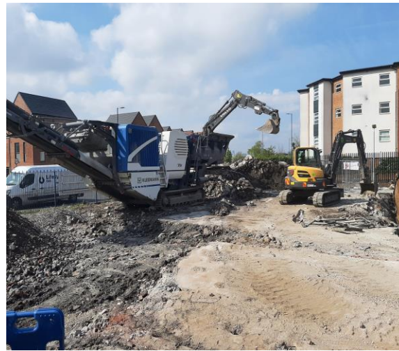
Image 11: Crushing works
