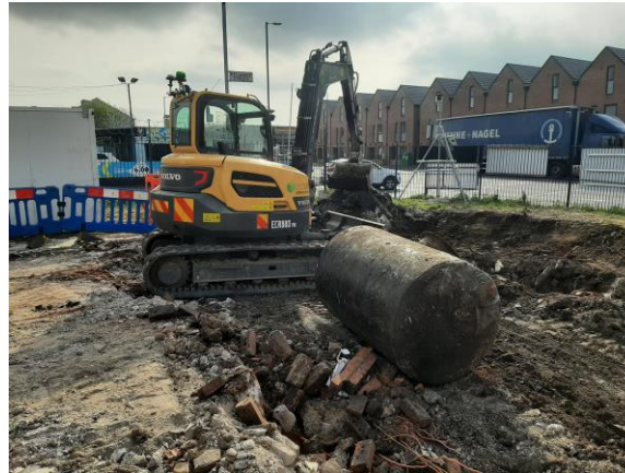
Image 11: Breaking out of interceptor
