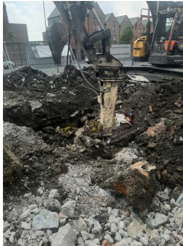
Image 11: Breaking out of interceptor
