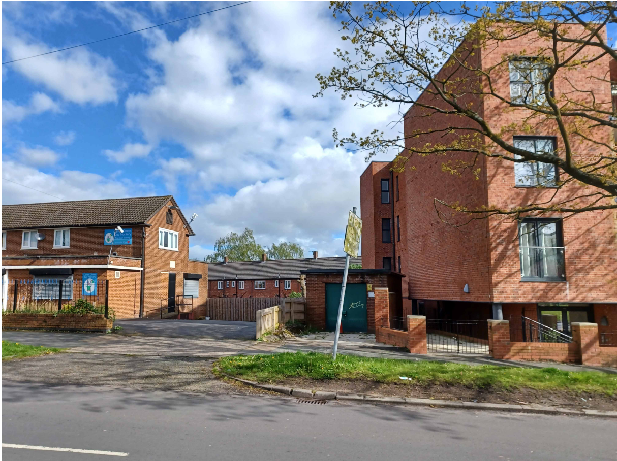
View north across the application site with the adjacent apartment building to the right
