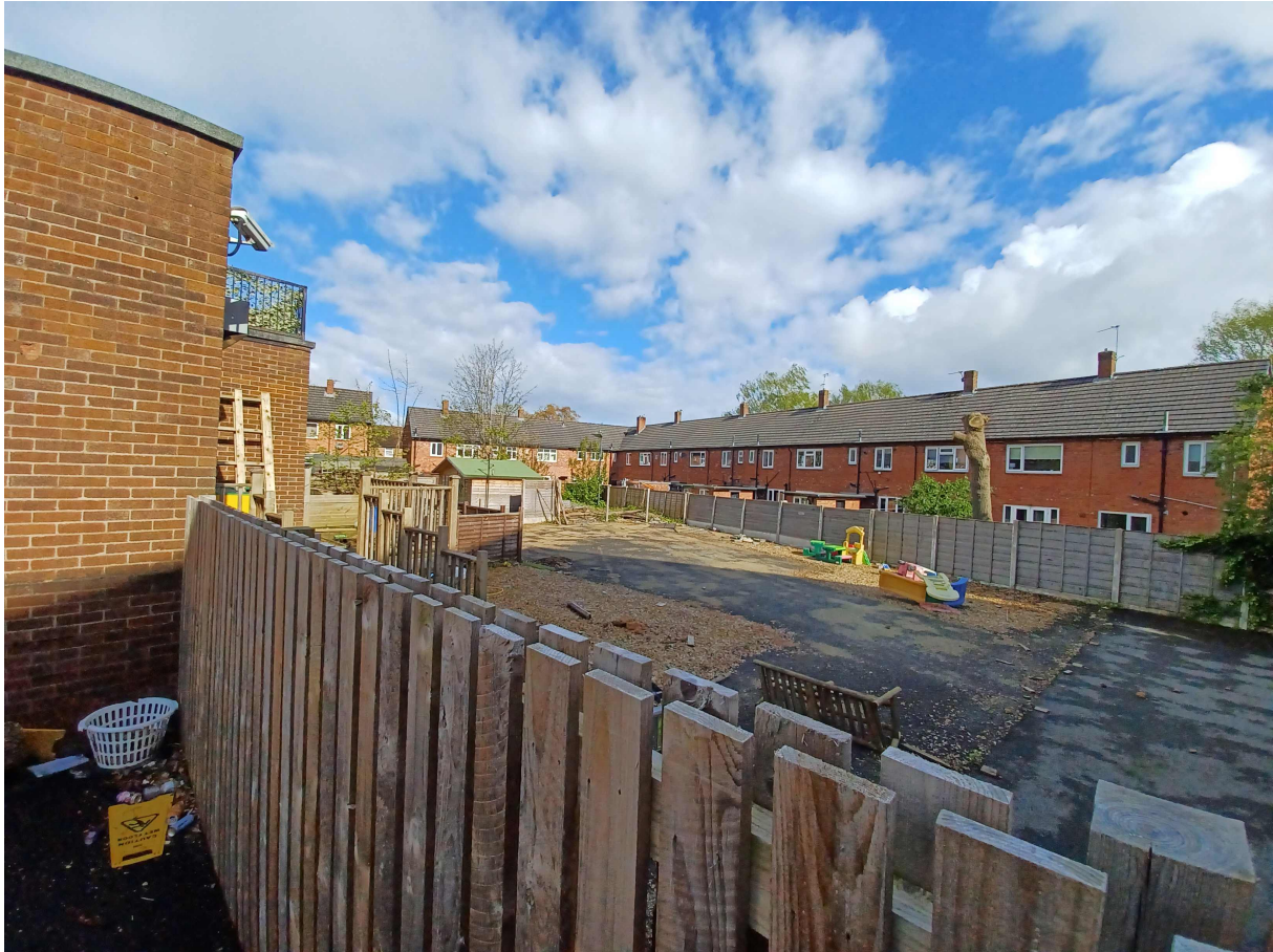
View across the rear of the site towards the rear of properties on Barnwood Road
