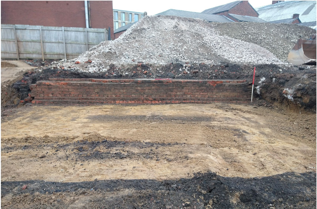
Plate 6: Western end of the north wall [004], looking north (scales = 1m)
