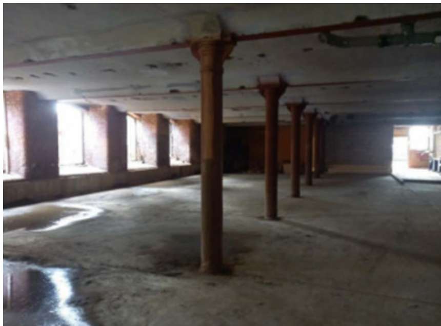
Image of basement area proposed to be converted
