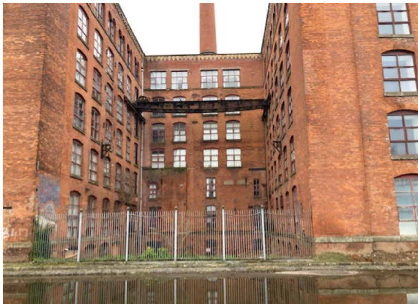
View of the mill from the opposite side of the Rochdale Canal
