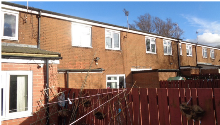
Rear Elevation of Adjacent Properties.
