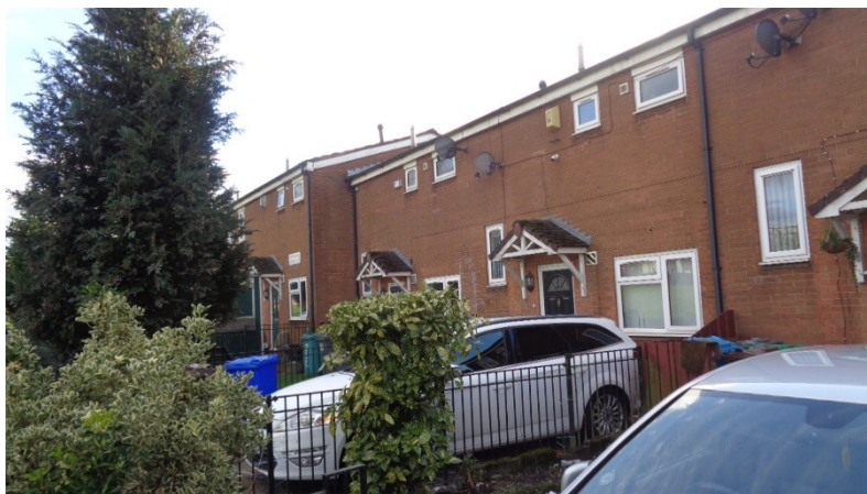
Front and Adjacent Elevations of Application Property.
