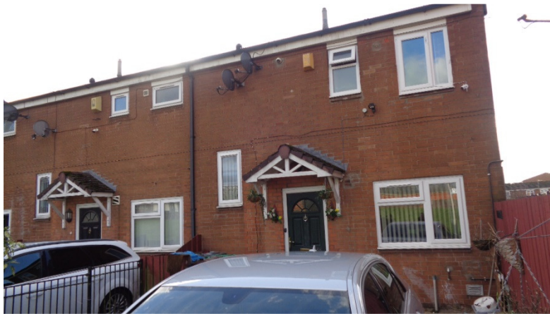
Front Elevation to Application Property.
