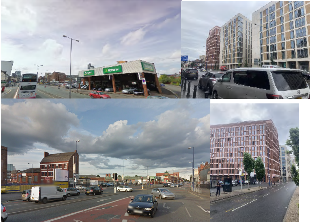
Figure 8. Showing frontage along Oldham Road in New Cross NDF Zone A. Left hand side shows situation in 2011 when application reference 095582/AOH/2011/N1 was submitted/ Right hand side shows situation as of August 2024. (Sources: Google Maps/ Author's own)
