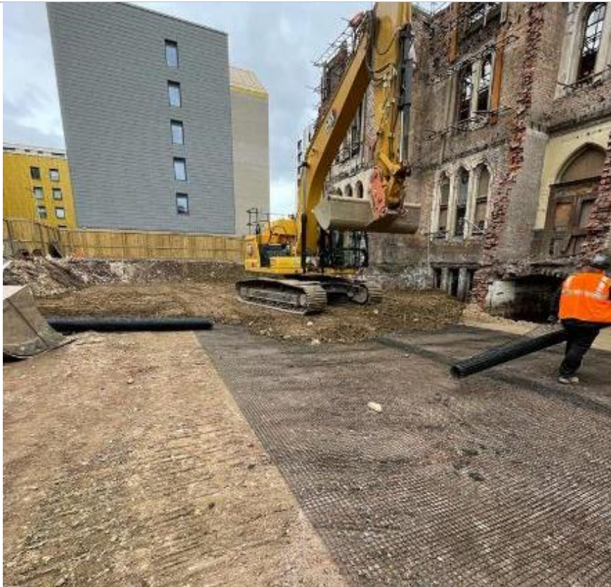
PLATE 4 23/05/2022 LAYING GEOTEXTILE ON UNDERLYING NATURAL GROUND AND INITIAL LAYER OF IMPORTED 6F2.
