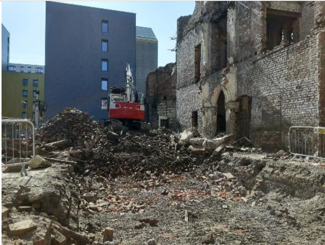
PLATE 2 22/04/2022 VIEW OF THE ONGOING DEMOLITION FACING WEST
