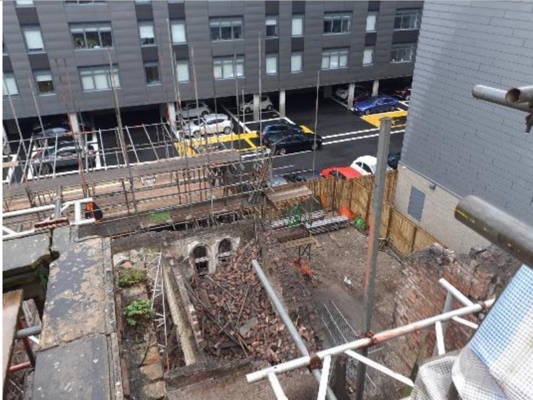
PLATE 1 04/04/2022 – VIEW OF PHASE 1 AREA PRIOR TO DEMOLITION
