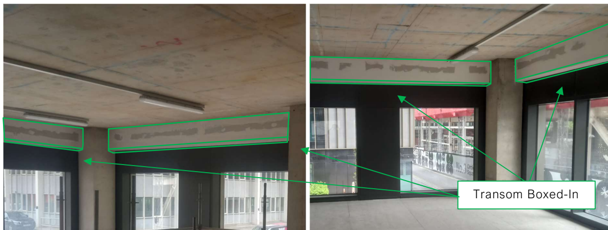
Figure 6 – On-site Curtain Wall Detailing
