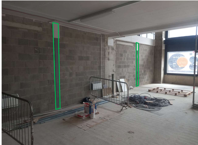
Figure 8 – Vertical Steel Detail Locations
