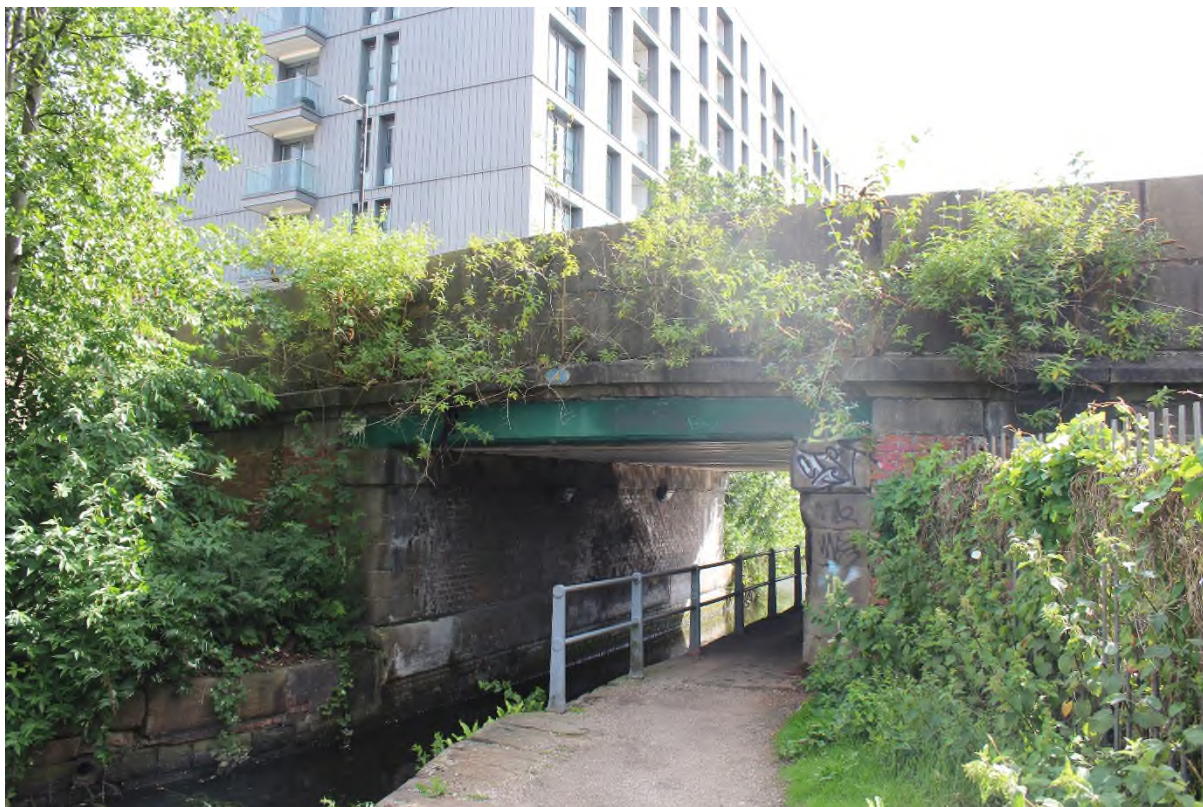
Figure 6-10 Bridge Number 4 Over Ashton Canal (Authors Own)
