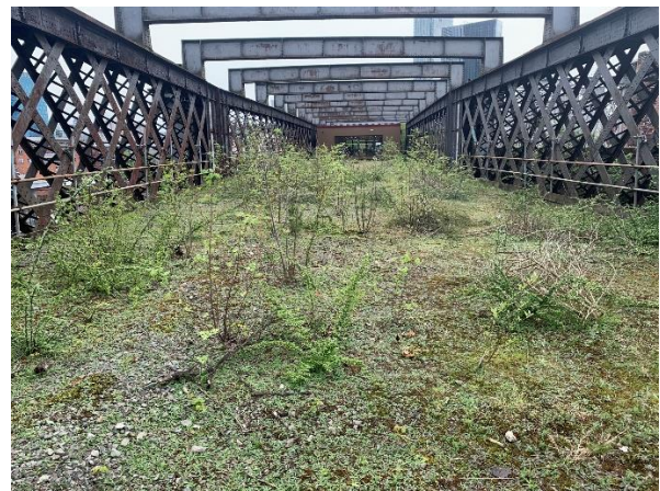
Photograph 11 – Sparsely vegetated section of viaduct
