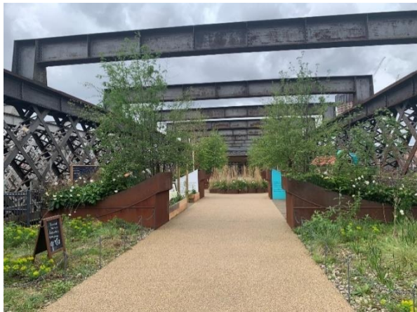
Photograph 1 – Path through centre of viaduct
