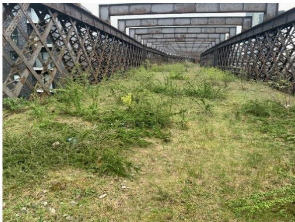
Photograph 10 – Sparsely vegetated section of viaduct
