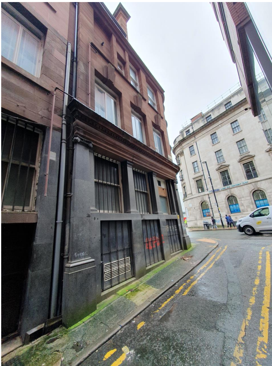
Figure 8: Rear Elevation existing louvres to lower ground and ground floor identified
