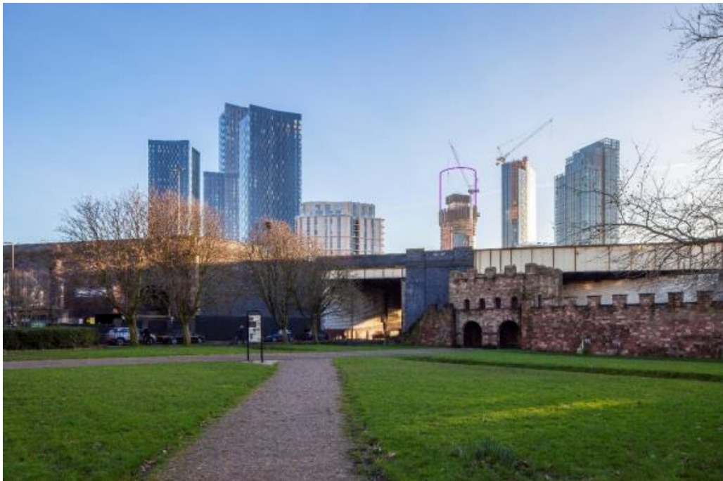
View 8 – Existing View from the Roman Fort, Castlefield
